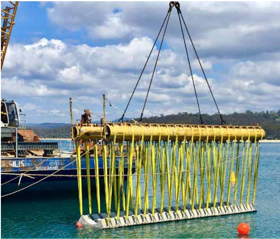
A section of scour protection being lowered into place in Eden recently.
