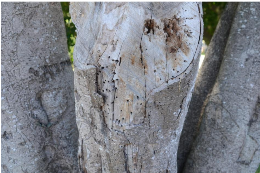
Figure 4; indication of insect attack found in the dead timber directly associated with pruning cut. The healthy wood of a living stem is able to resist borer attack however, as die-back occurs and vitality drops these predators are able to gain access.
