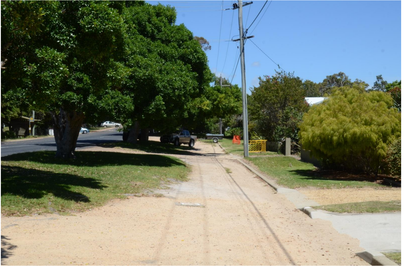
Figure 1; View of trees 11 and 12 showing the typical canopy spread. Note the proximity of high voltage conductors that will require future pruning as the canopy enters clearance zones.
