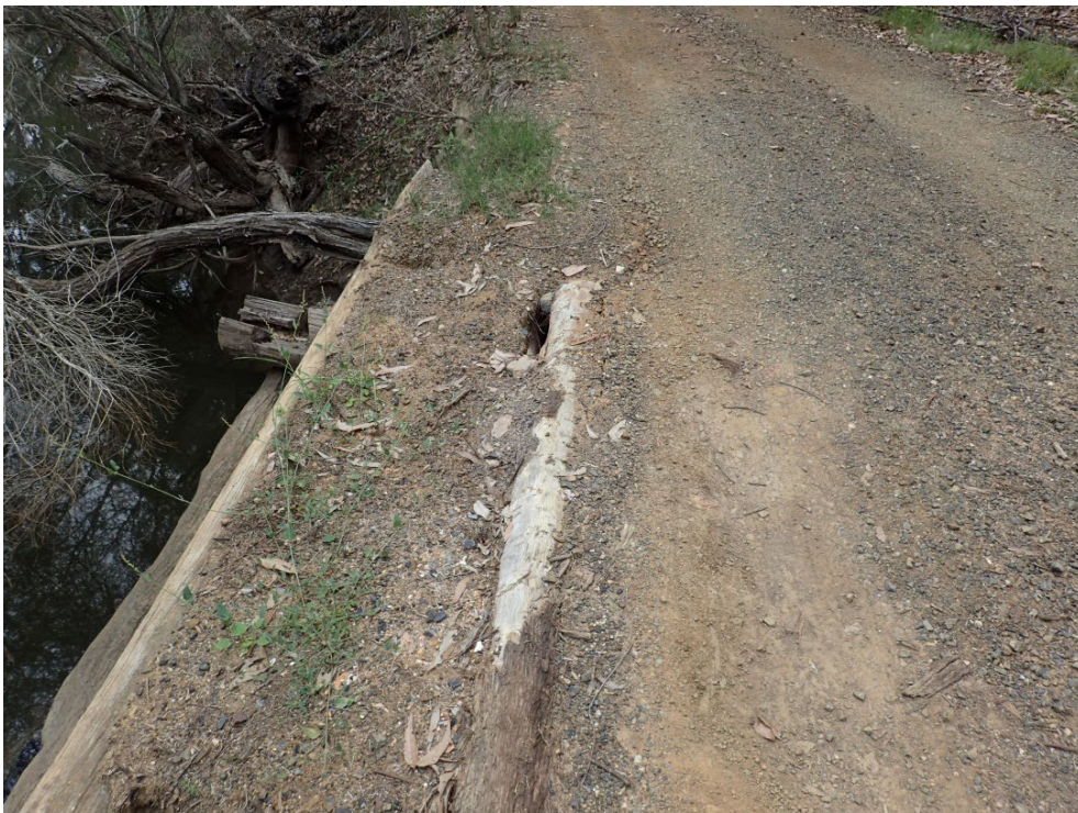
Figure 8: Log bridge on Scenic Forest Way, across Black Lagoon
