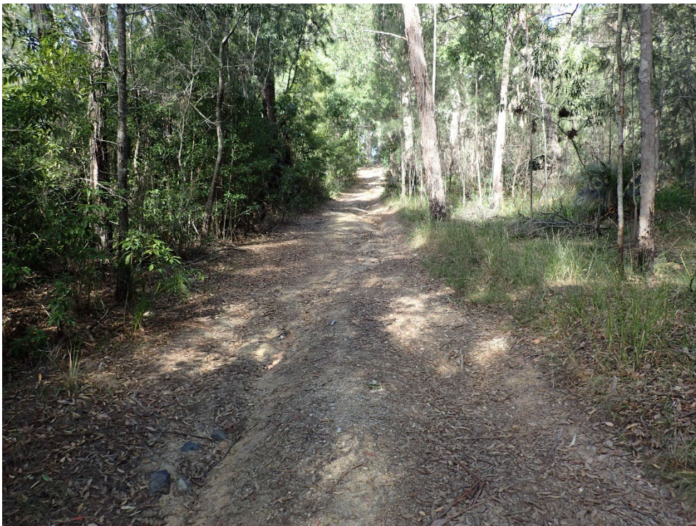
Figure 7: Poor condition unsealed track
