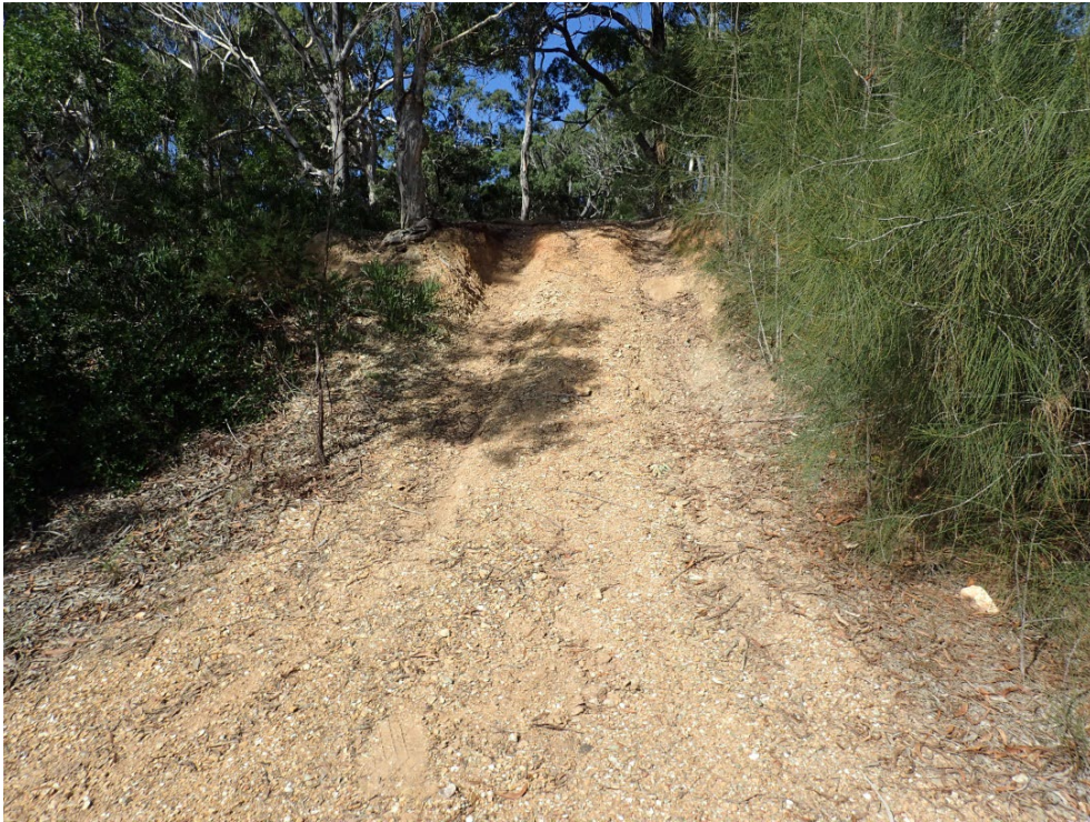
Figure 6: Eroding surface of former vehicle track
