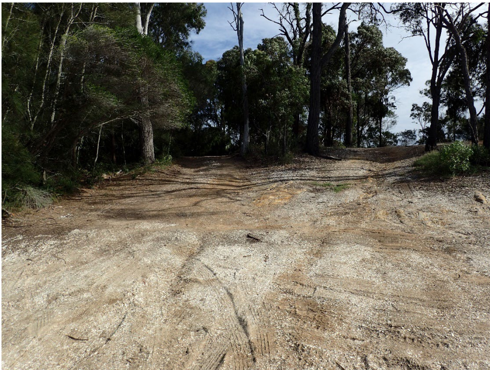
Figure 5: Eroding surface of former vehicle turning area, Fairhaven Point Way
