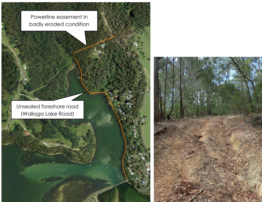
Figure 1: Unsealed foreshore road and eroded powerline easement track at Akolele
