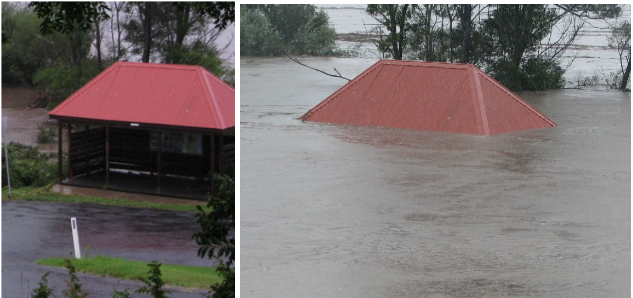
Figure 5-3 Towamba Bus Shelter Flooding in 2011
