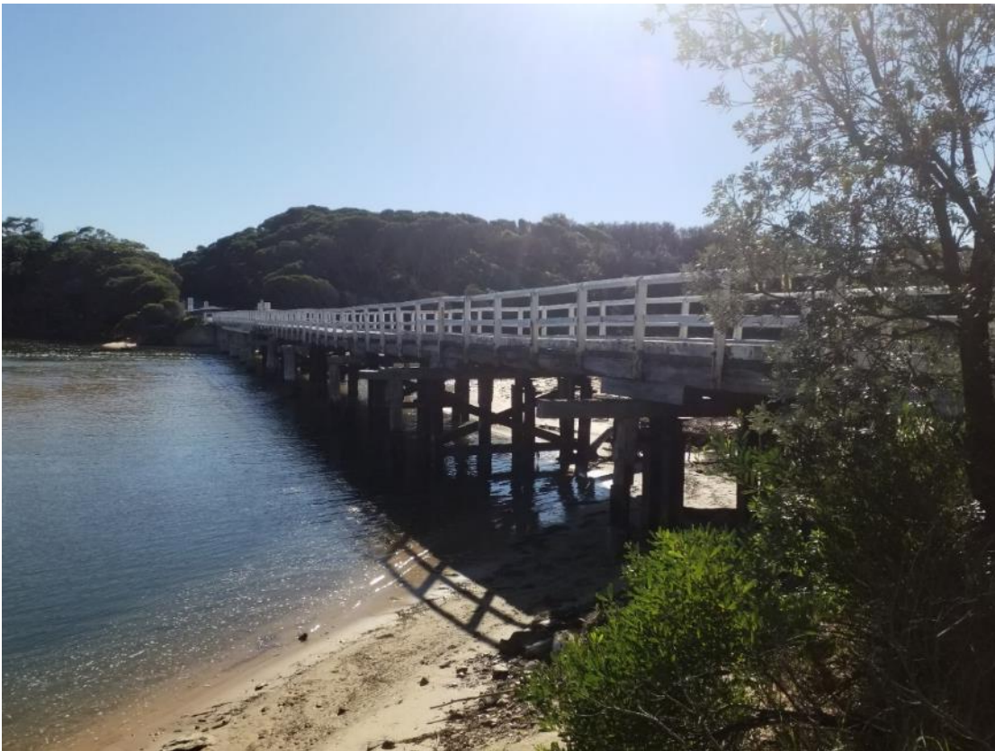
Figure 2-4 Cuttagee Creek Bridge
