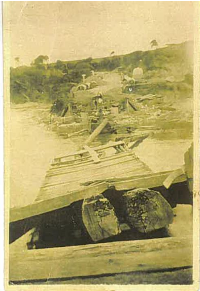
Cuttagee bridge looking north from about pier 4 showing demolition of the northern end of the bridge circa 1934-35. Source Murrah Hall Committee.
