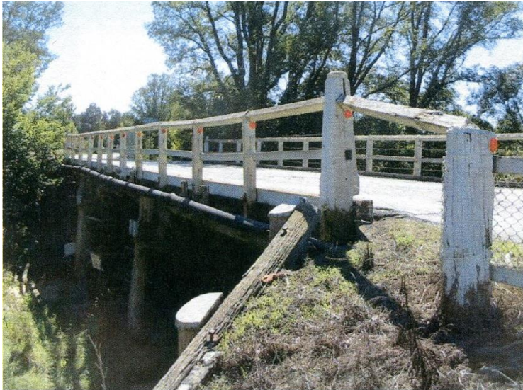
Turallo Creek, Bungendore (Palerang Shire), prior to demolition
