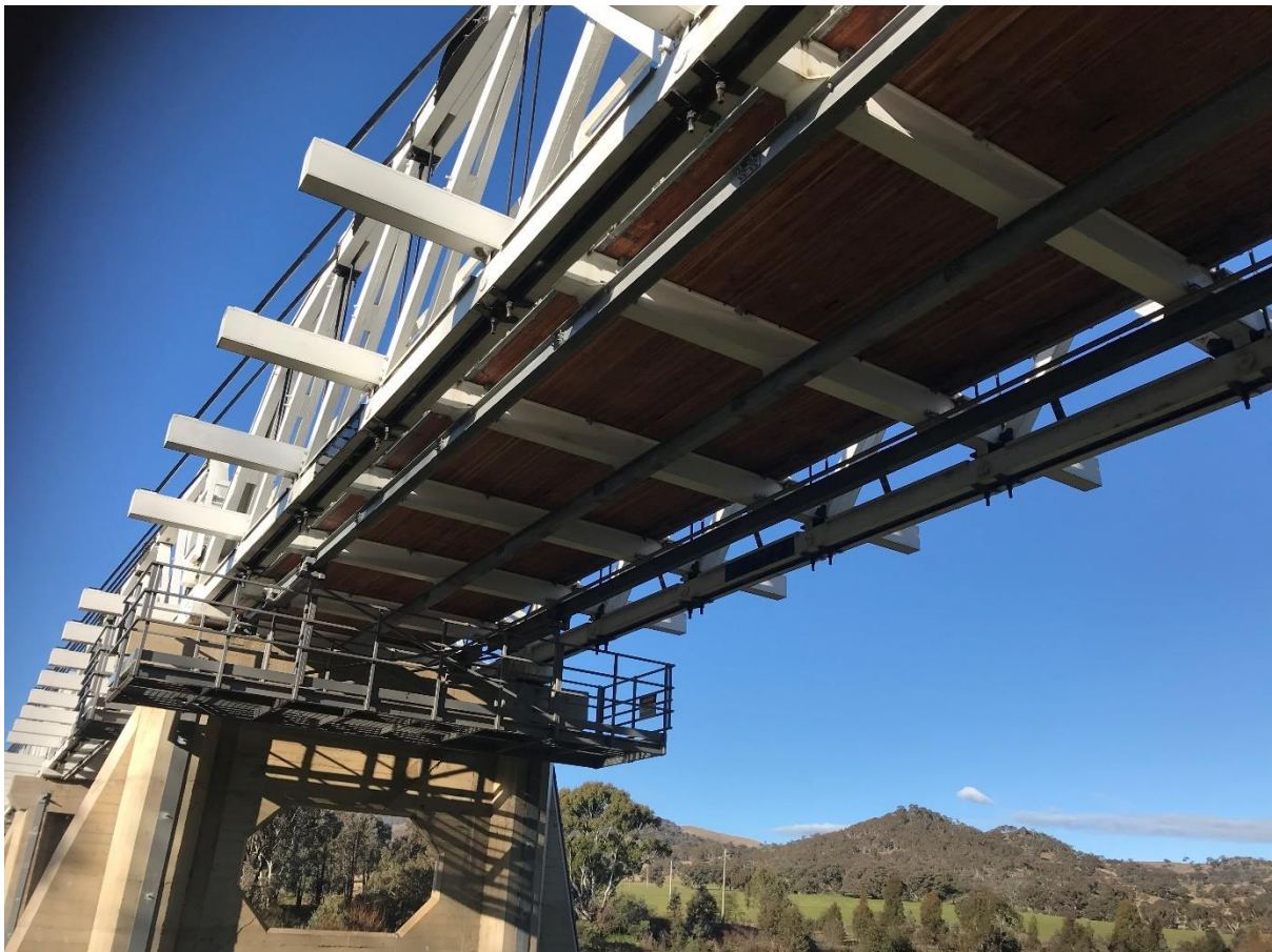
The welded steel cross-beams support the laminated timber deck. Photo July 2021.
