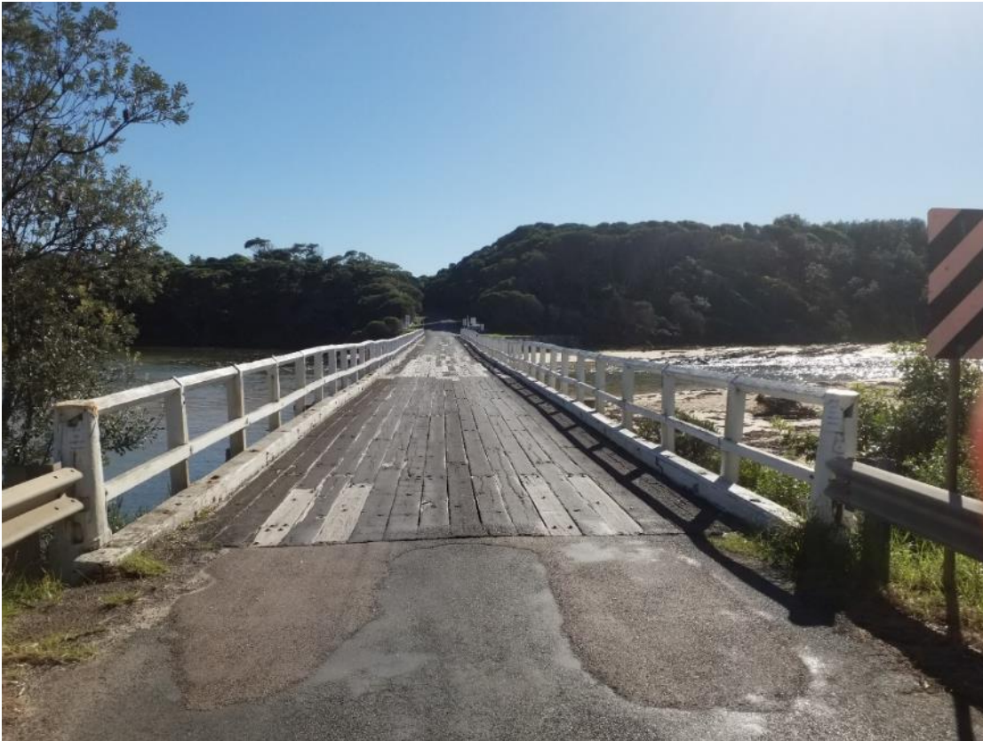
Figure 2-3 Cuttagee Creek Bridge (looking north)
