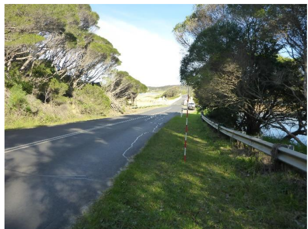
Plate 2 View south from north side of bridge, note existing disturbance.
