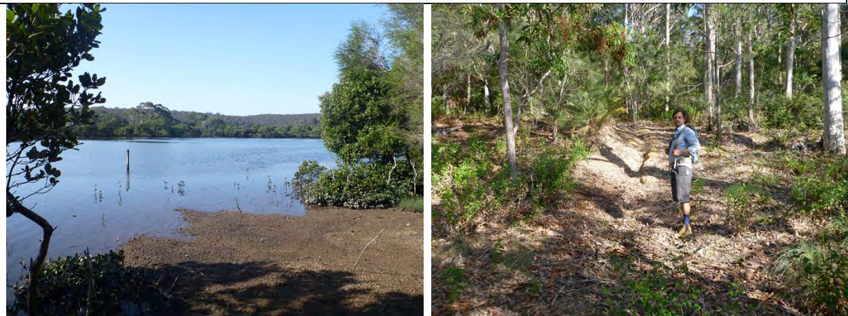
Figure B21 Deposition of hill slope sediments at the margin of estuary back lagoon due to erosion of old foreshore access track ( left image ). Example of erosion affecting the foreshore access track ( right image ).
