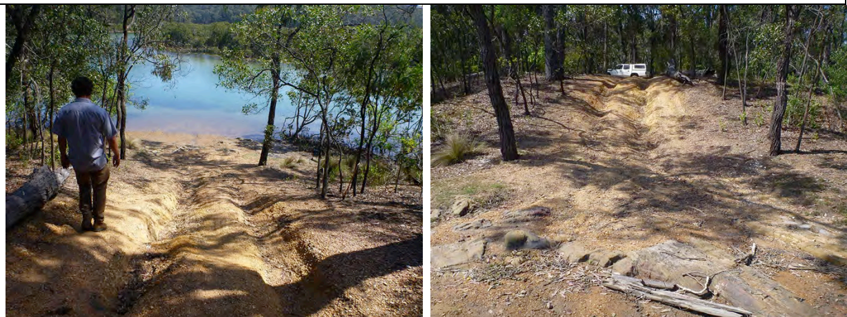
Figure B12. Vehicle access to the foreshore from Cowdroys road with moderate erosion and wheel rutting evident ( left image ). Current road condition is relatively stable with majority of dispersible sediment already eroded ( right image ).
