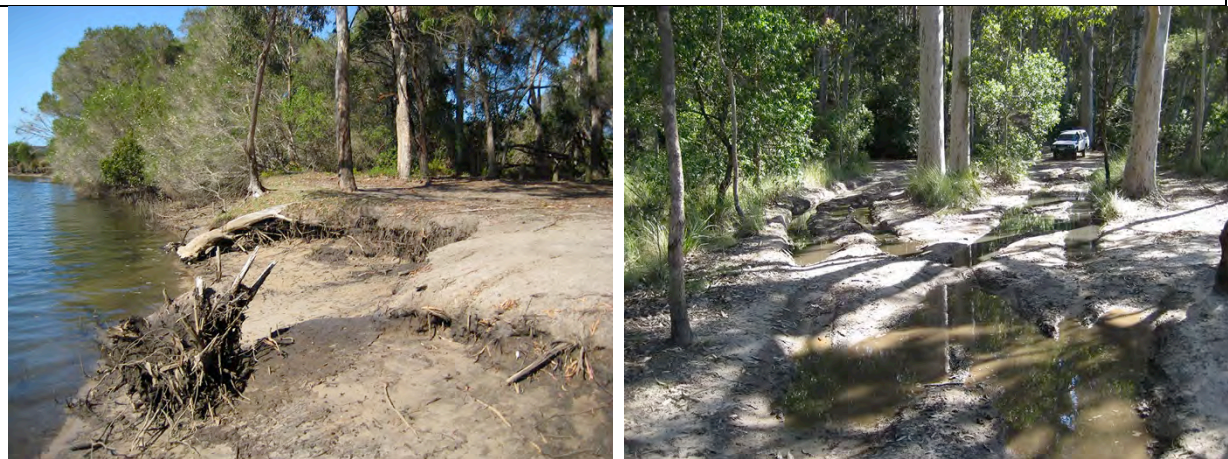
Figure B9 Degraded bank currently devoid of any regenerating vegetation ( left image ). Parts of the foreshore access road are in poor condition with deep wheel ruts and mud tracks ( right image ).
