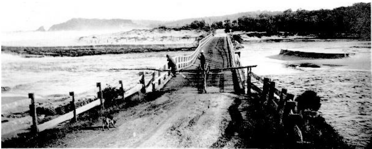
Cuttagee bridge looking south following collapse of spans 2 and 3 during heavy storms in 1934.
