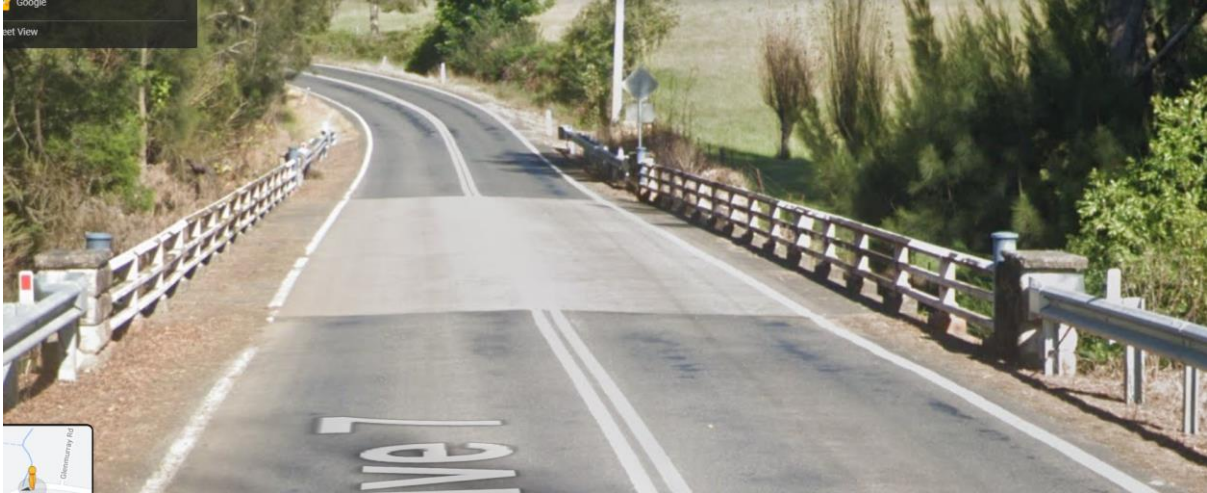
Glenmurray bridge sits well within its context. Google Image of 2021
