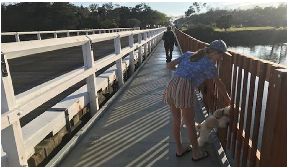
The historic timber railings on the vehicle bridge have been upgraded and painted. The balustrade on the pedestrian bridge has also been upgraded by changing from galvanised steel pipe to clear finished timber.
