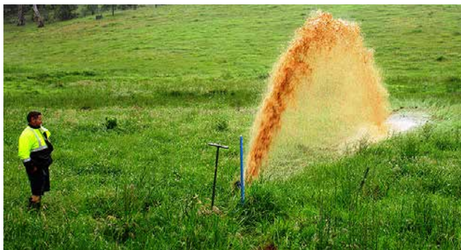
Bega Water and Sewer Services team member, Scott Reeve, flushing the water main between Bega and Tathra in 2015.
