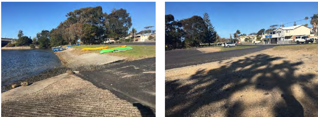
Figure 2-1 Existing infrastructure and facilities at the Bermagui River boat ramp precinct.
