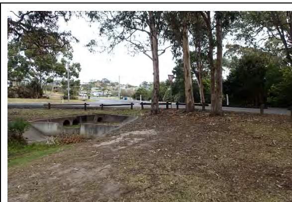
Plate 9. View west to road intersection showing built up roadway and underground stormwater drainage structures.
