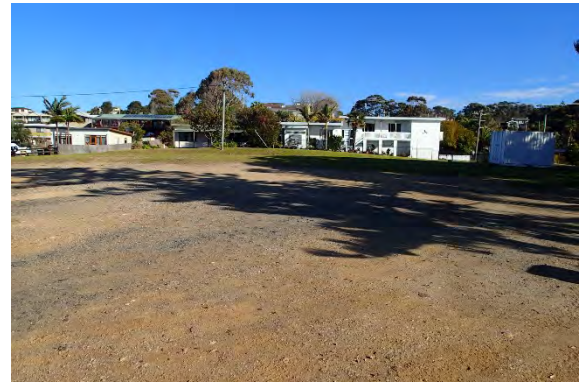
Plate 2. View south to large eroded carpark extension.
