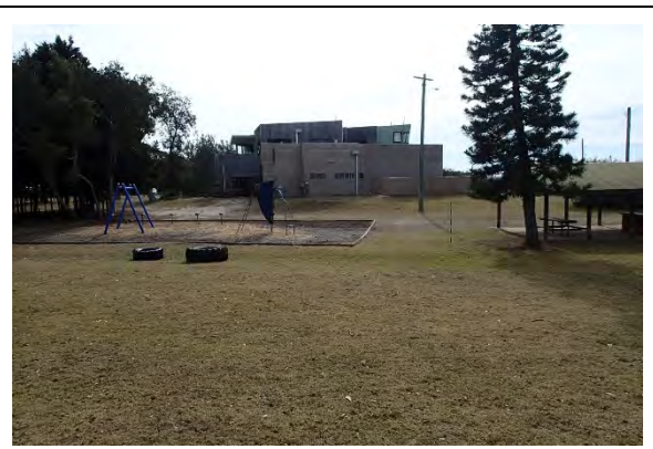
Plate 10. View north across existing facilities to club, note some exposures and planted conifers on left.
