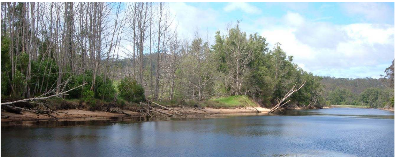
Figure 2-6 Bank Erosion: Site B (refer Figure B-8)
