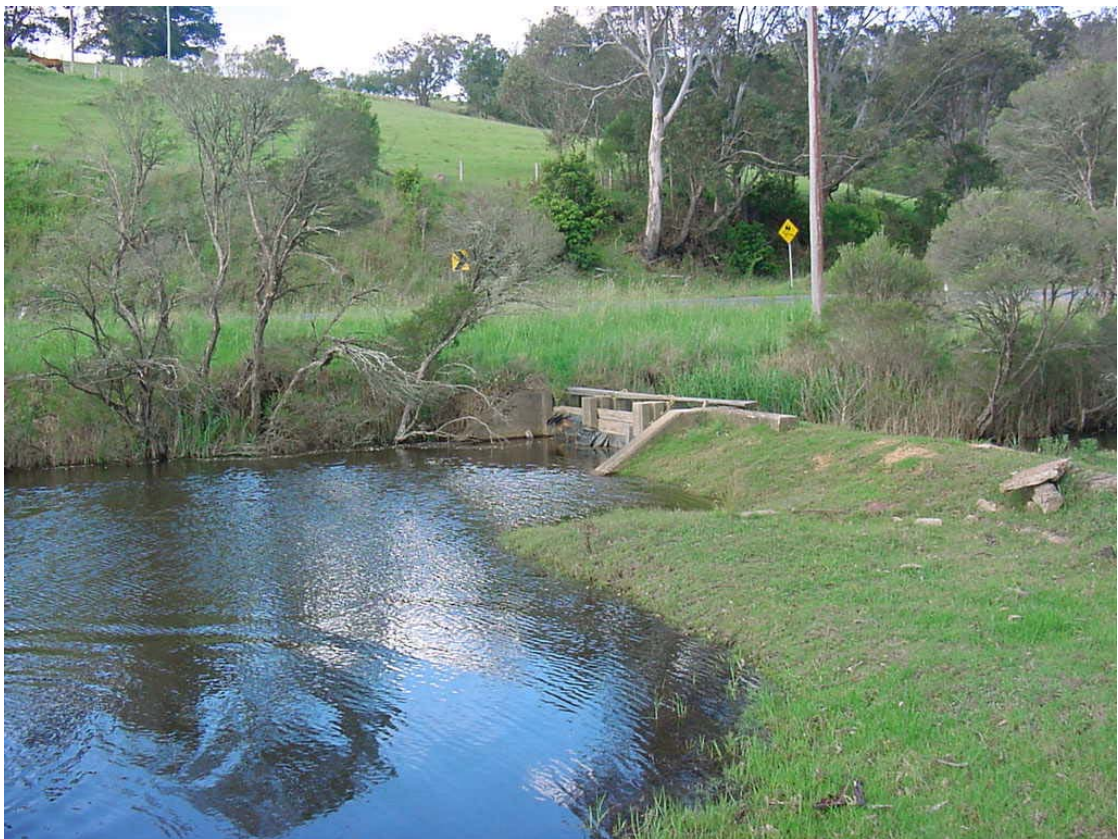
Figure 2-4 The original Russell Creek Weir when downstream water levels are low (top photo: Nov. 05) and high (bottom photo: Nov. 04) (high water levels as the result of a closed ocean entrance)
