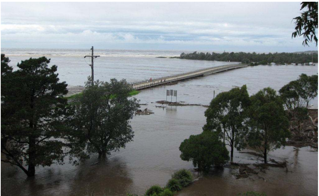
Figure 2-2 Hancock Bridge and Bega River entrance, March 2011 flood event
