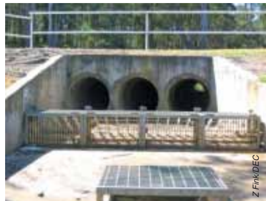
Gross pollutant trap on pipes upstream of the scheme
