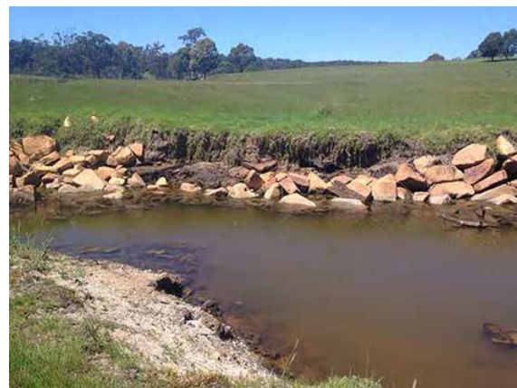
Figure B12 Large granite boulders placed at the culvert outlet for bed protection ( left image ). The
