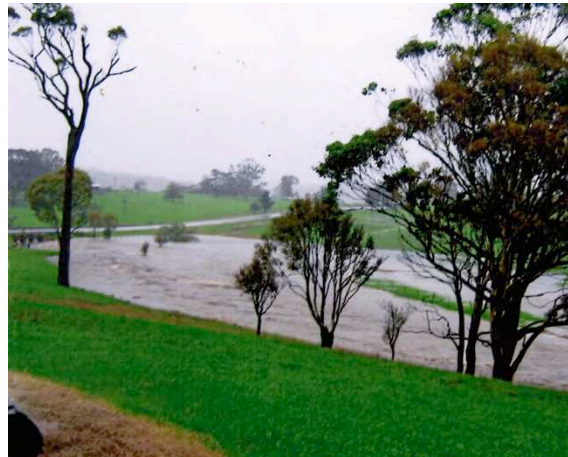
Figure B16 Example of how the road embankment acts like a dam wall causing floodwaters to build-up on the western side of Tathra-Bermagui Road ( photos courtesy of N. Dummett, 15 February 2010 ).
