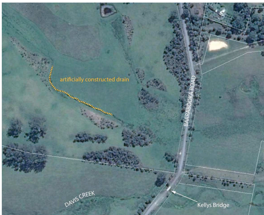
Figure B32 Location of an artificially constructed drain through a floodplain wetland that is now undergoing rehabilitation works.
