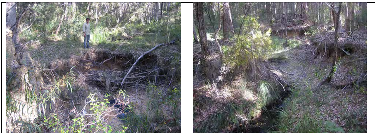
Figure 18. Example of active head cut in forested setting of Sandy Creek sub-catchment.
