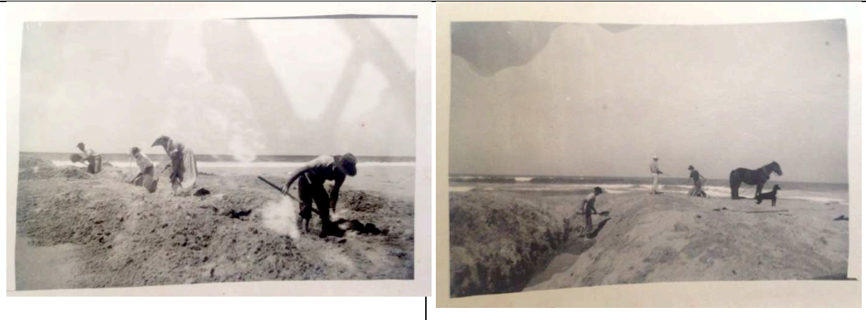
Figure B25. Historical management of the Middle Lagoon ocean entrance – circa 1950s (photos courtesy of N. Dummett).
