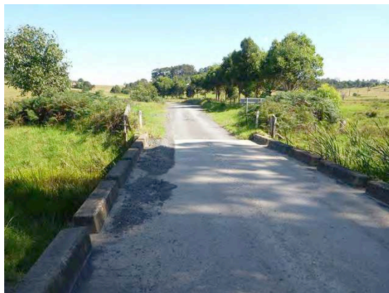
Figure B31 Gravel deposits transported to Kellys Bridge from Barrabooka road surface runoff after recent heavy rainfall event ( left image ). Gravel deposits accumulating in roadside drain adjacent to
