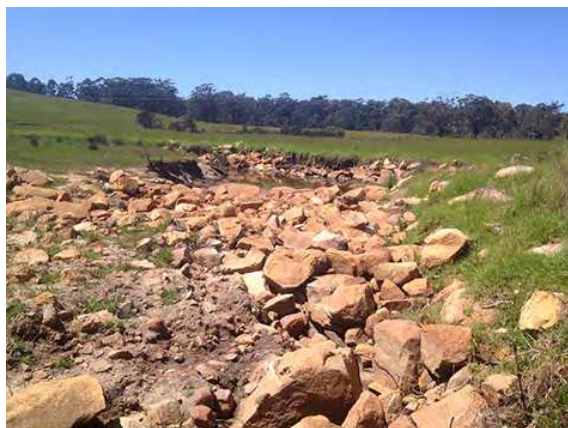
Figure B12 Large granite boulders placed at the culvert outlet for bed protection ( left image ). The
