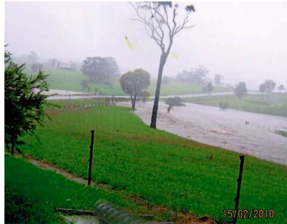
Figure B16 Example of how the road embankment acts like a dam wall causing floodwaters to build-up on the western side of Tathra-Bermagui Road ( photos courtesy of N. Dummett, 15 February 2010 ).
