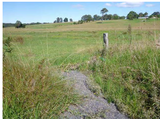
Figure B31 Gravel deposits transported to Kellys Bridge from Barrabooka road surface runoff after recent heavy rainfall event ( left image ). Gravel deposits accumulating in roadside drain adjacent to
