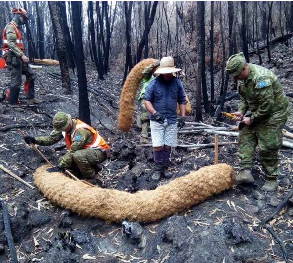
Erosion sediment controls being deployed in Wonboyn, with Local contractors including Paddy Farrell and Creative Lines, with assistance from Australian Defence Force members.
