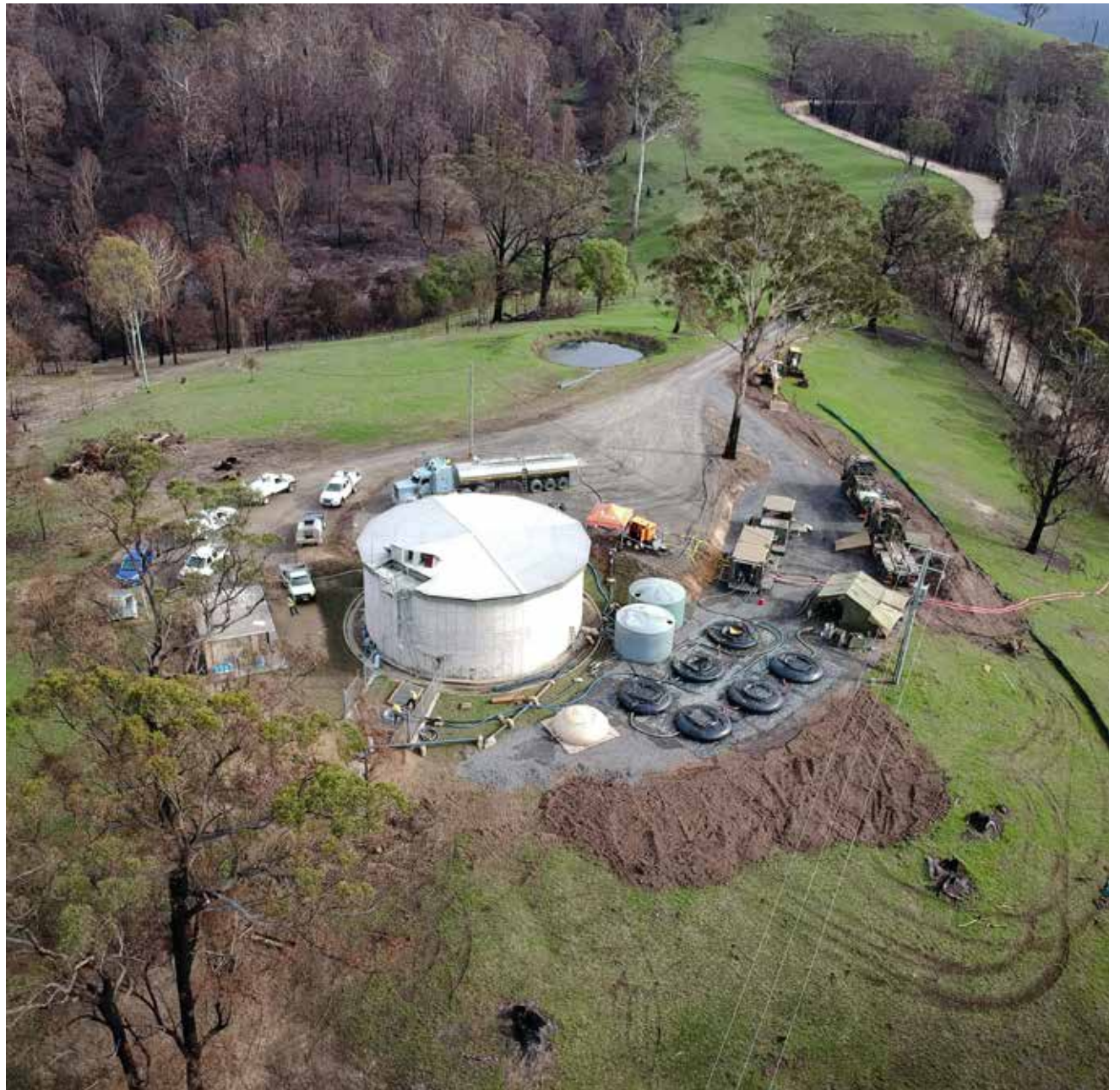
The ADF have set up a water purification and desalination system (WPDS) next to Brogo Tank One to help supplement the drinking water supplies.
