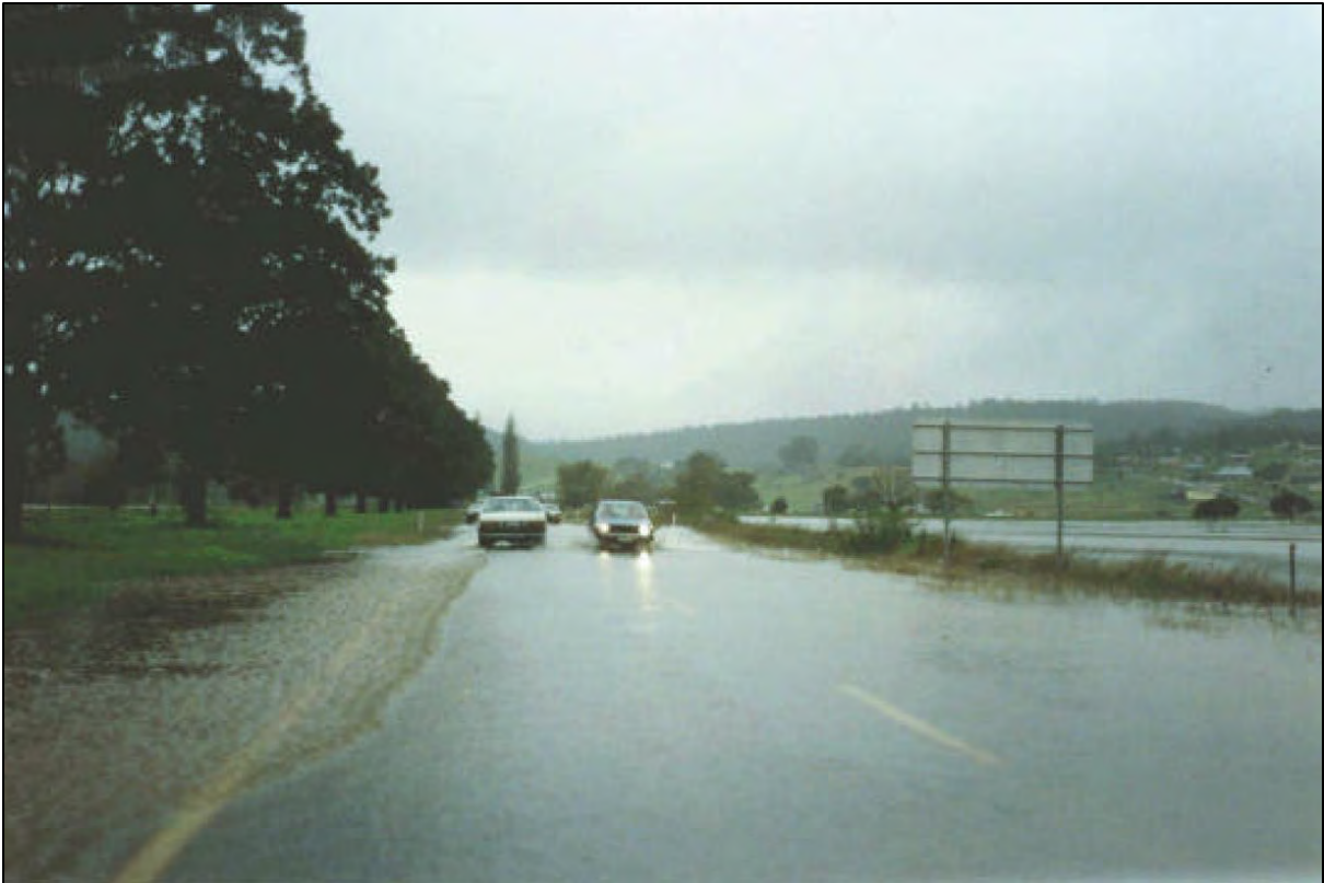
Plate 4 View looking south along Princes Highway during 1990 flood (RTA, 2004)
