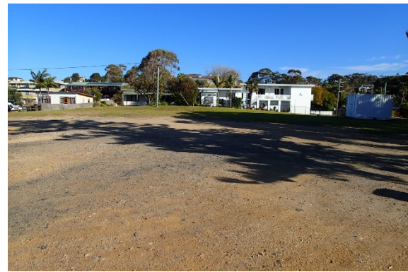
Plate 2. View south to large eroded carpark extension.
