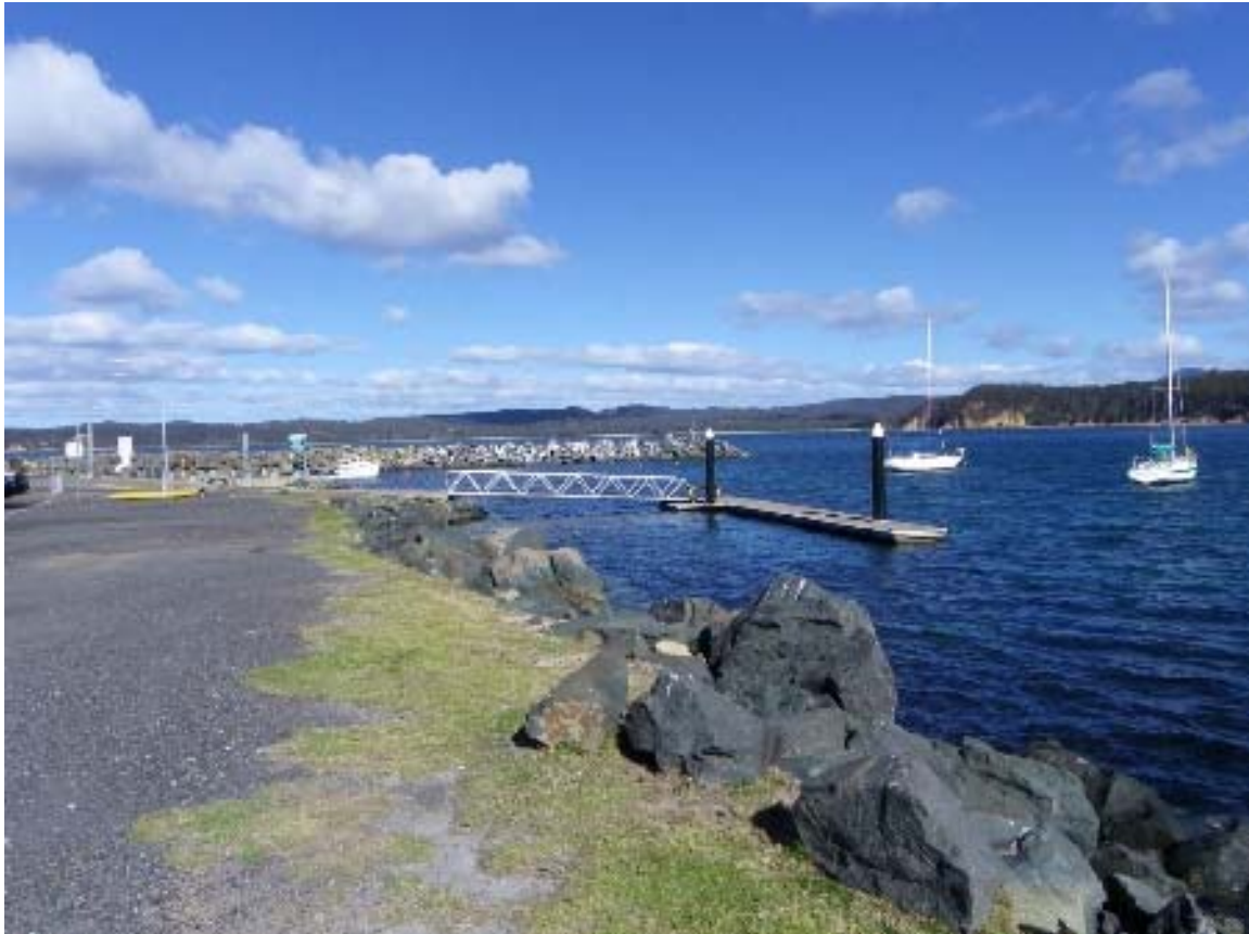
Figure 2-1 Existing finger pontoon jetty at Quarantine Bay.
