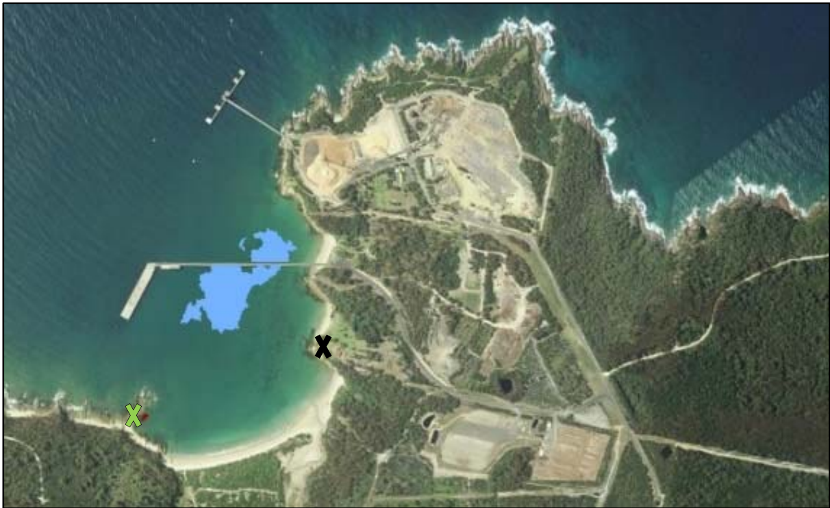
Figure 5-2 Distribution of mapped seagrass in relation to site (green X) and Edrom Lodge (black X) at the south end of Twofold Bay.
