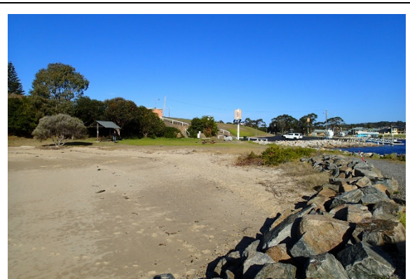
Plate 4. View south east across sand flat to natural bank showing existing path and toilet block. Note the carpark and sand flat are not natural.
