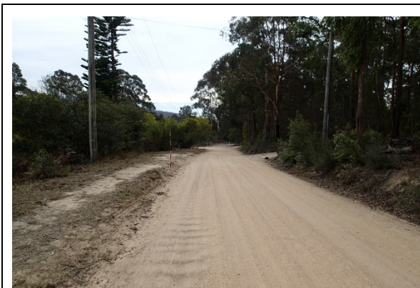
Plate 5. View north along road showing cutting and imported road base.
