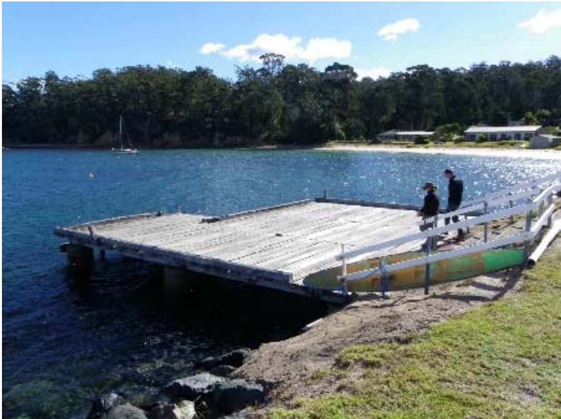
Figure 2-2 Existing stepped timber jetty at Quarantine Bay.
