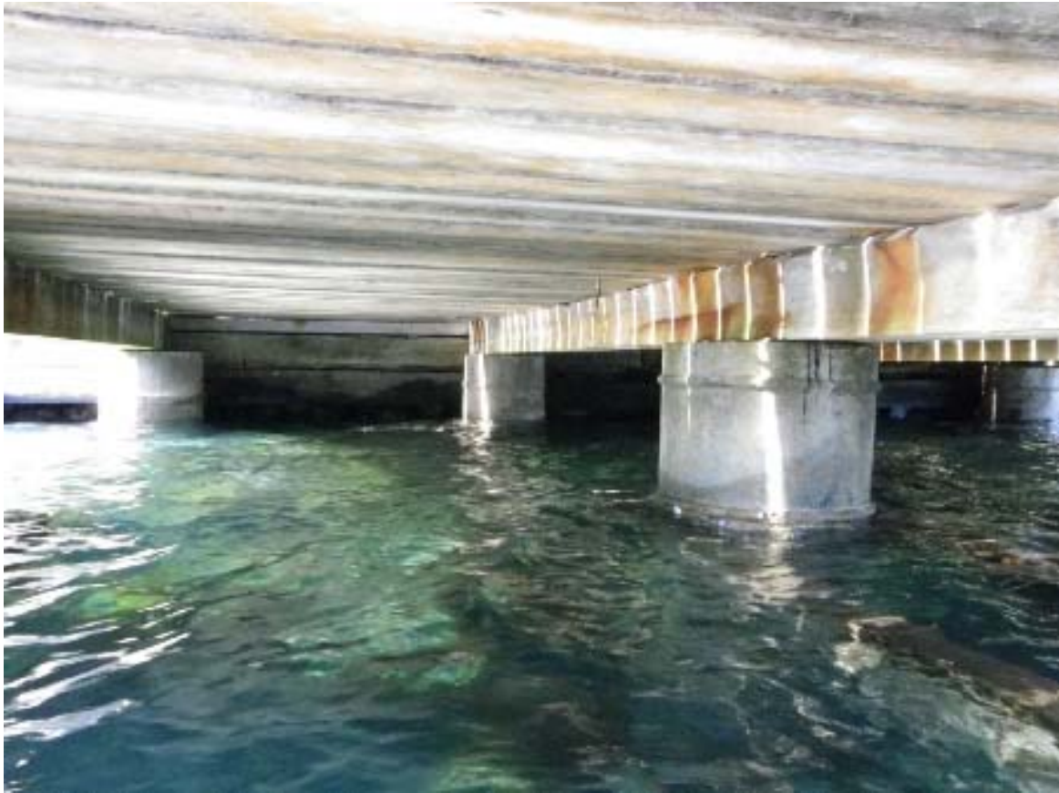
Figure 2-3 Existing stepped timber jetty at Quarantine Bay.
