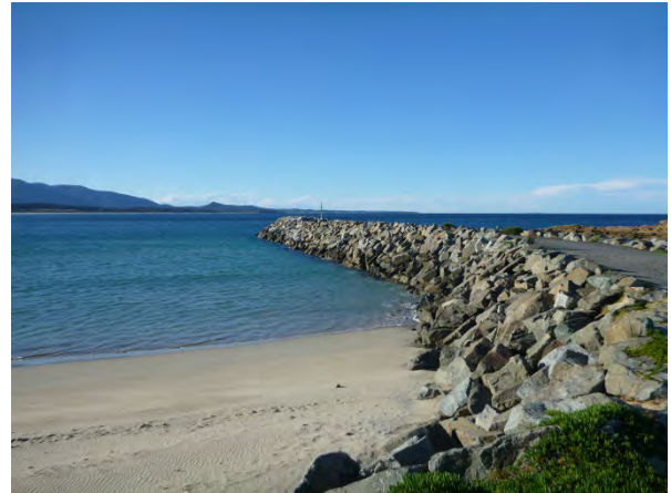
Bermagui River Training Walls
