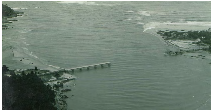
Figure 4-7 Hancock Bridge after February 1971 flood event (Image: O. Hinde)
