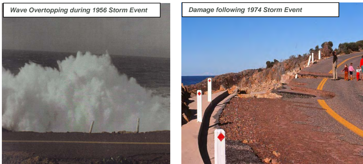
Figure 2-12 Wave Overtopping at Tathra Headland
