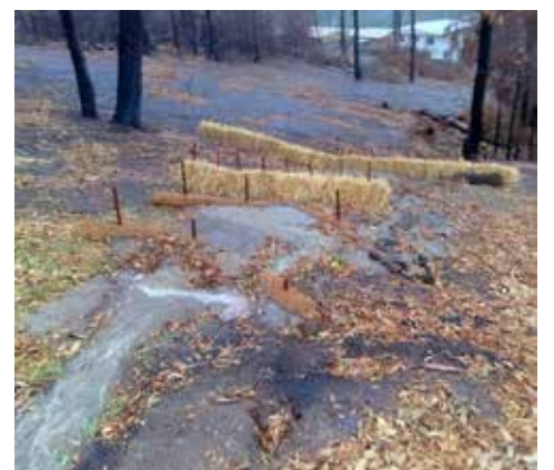
Hay bales and coir logs trapping stormwater and sediment during a recent rain event.
