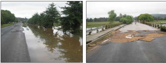
Flooding at Tarranganda Lane - 23 March 2011
