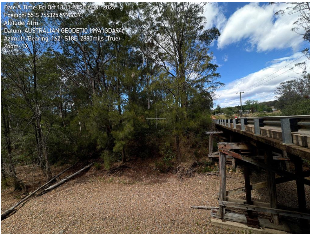
Photo 4, Alignment of proposed bridge facing south, vegetation in centre of image will be impacted.
