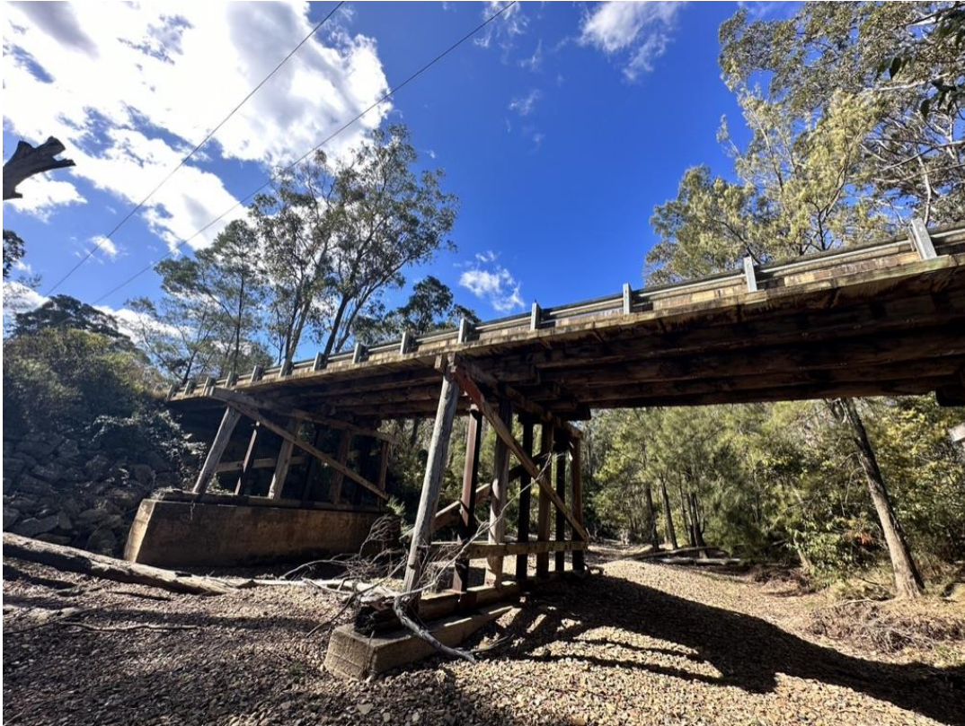
Photo 1, Existing Bridge from western side.
