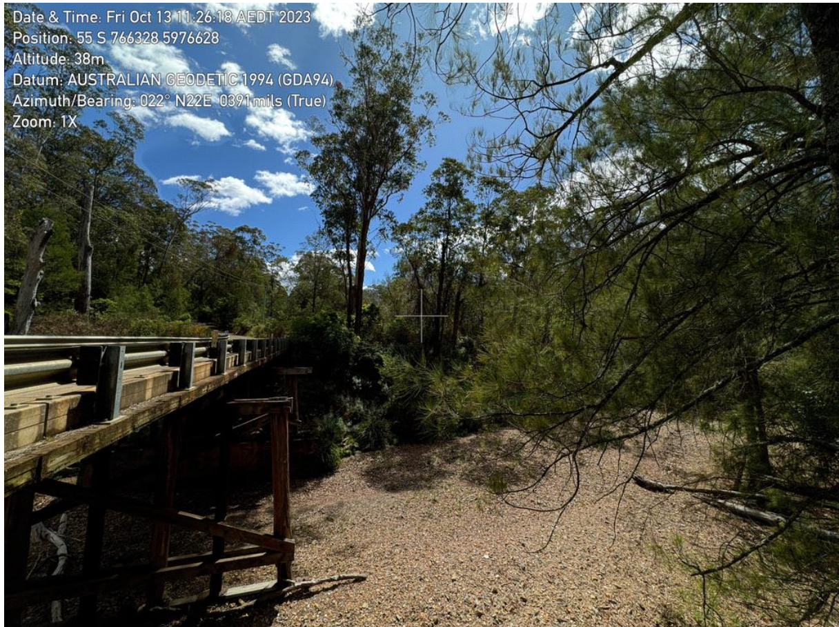
Photo 5, Alignment of proposed bridge facing north, vegetation in centre of image will be impacted.
