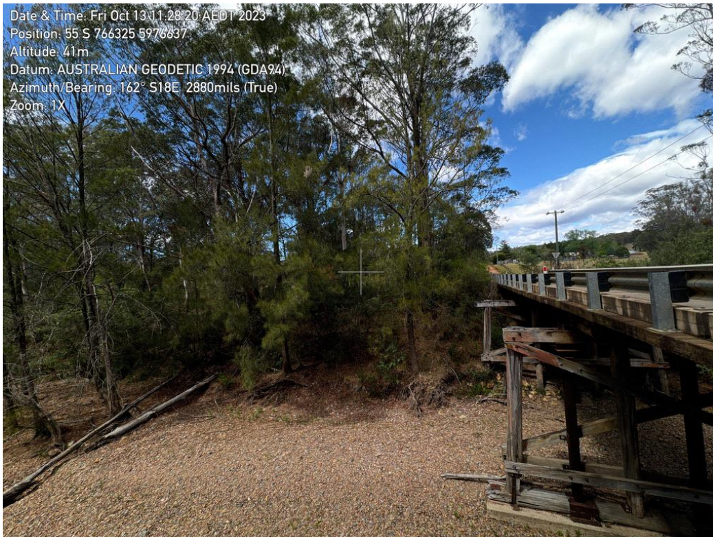
Photo 4, Alignment of proposed bridge facing south, vegetation in middle of image will be removed.
