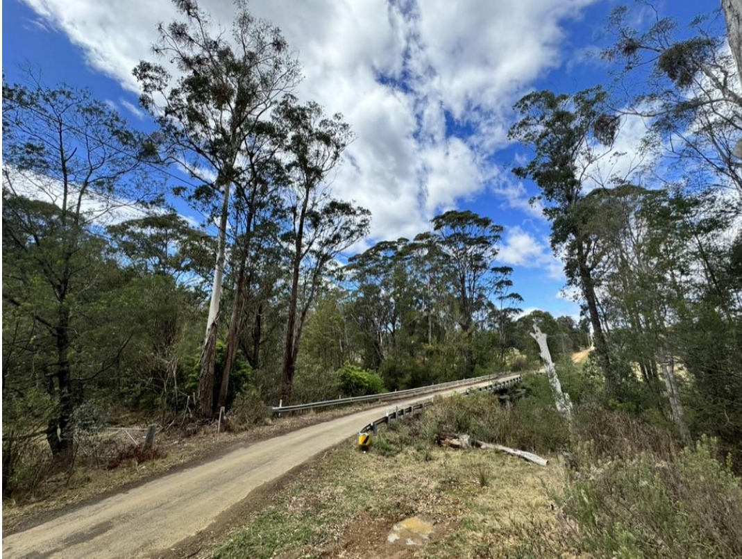
Photo 3, Existing Bridge from north side.
