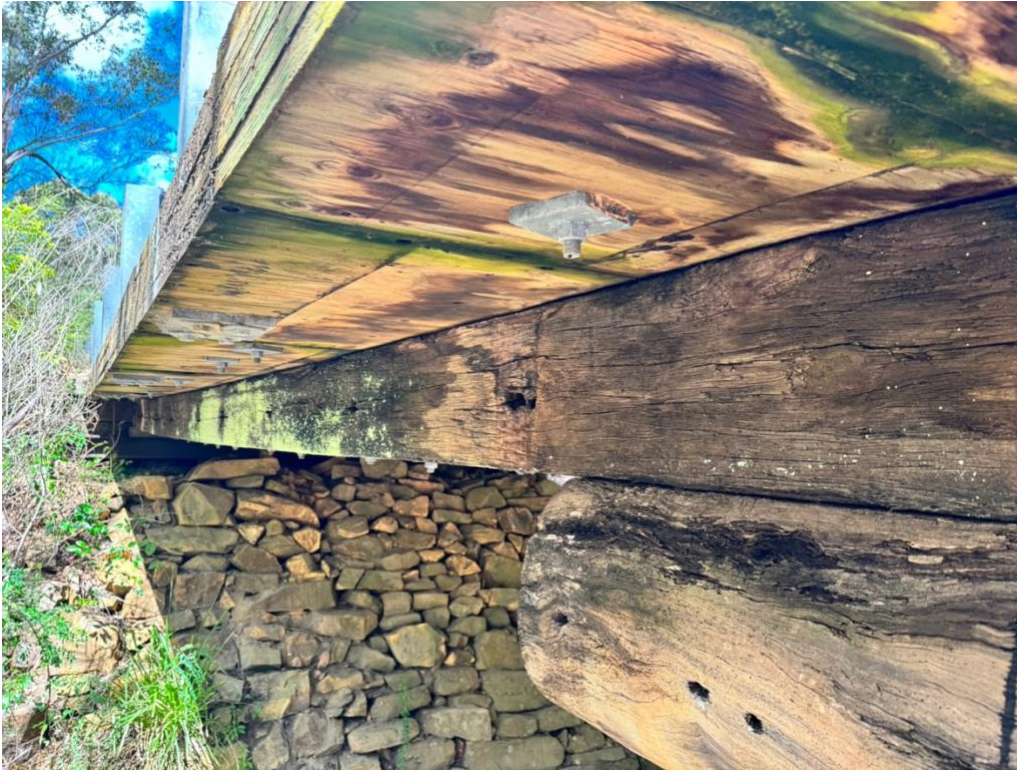
Figure 3-7, Rocky abutment/ scour protection on southern bank providing abundant refuge habitat particularly for insects, reptiles and small mammals.
