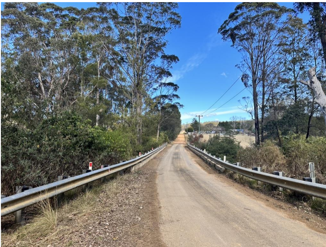
Photo 2, Existing Bridge from north side, proposed new bridge alignment is on the left hand side
