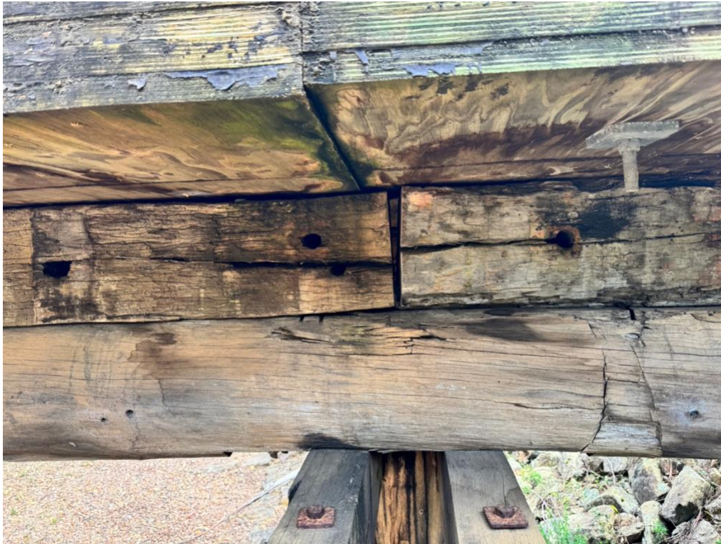
Figure 3-6, Examples of fissures in timber and cracks at timber joints that provide refuge and roosting habitat for a range of fauna particularly microbats.
