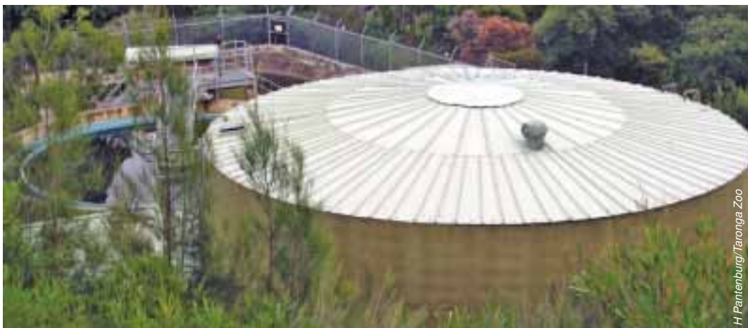
Taronga Zoo stormwater and wastewater treatment plant
