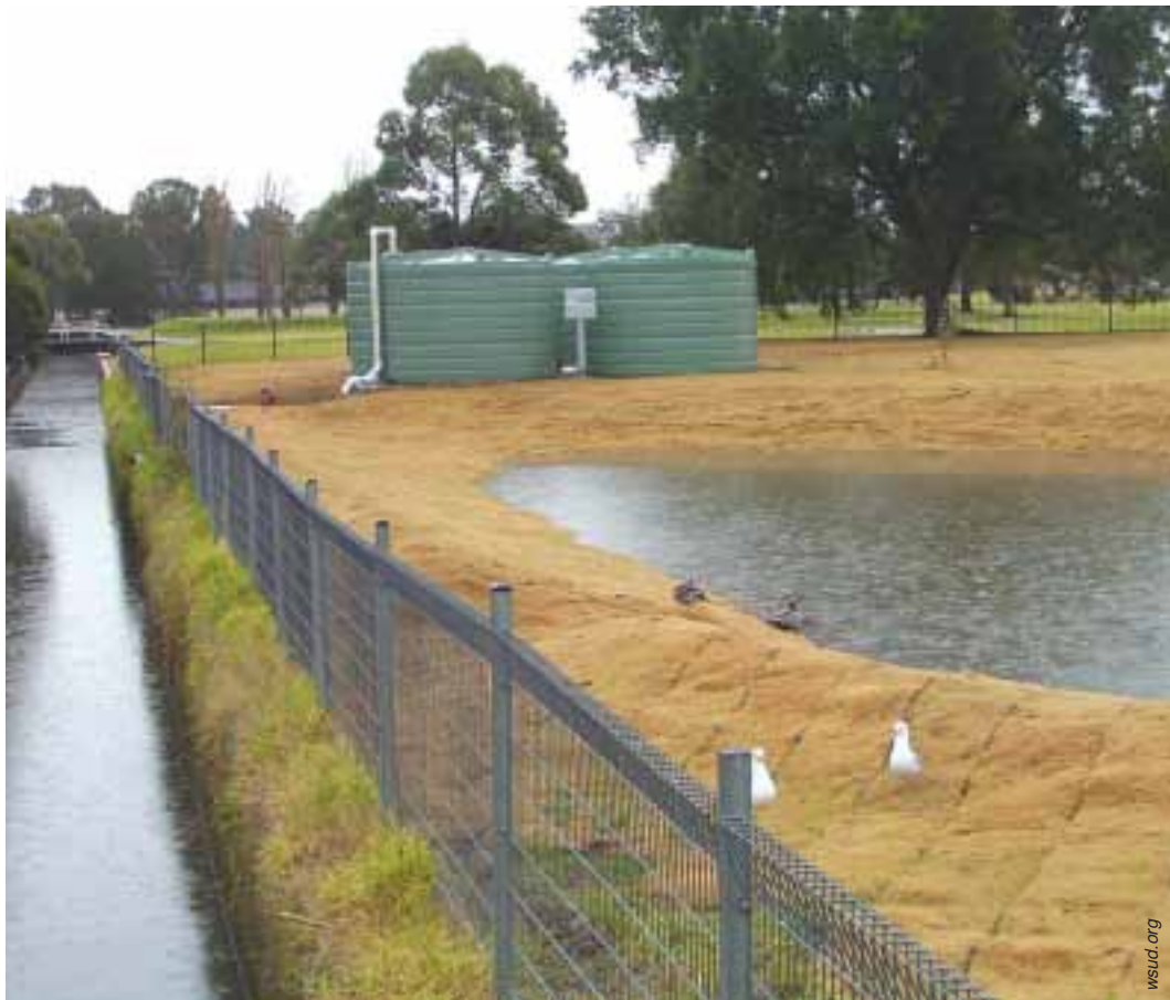
Barnwell Park Golf Course – stormwater channel, retention basins and storage tanks
