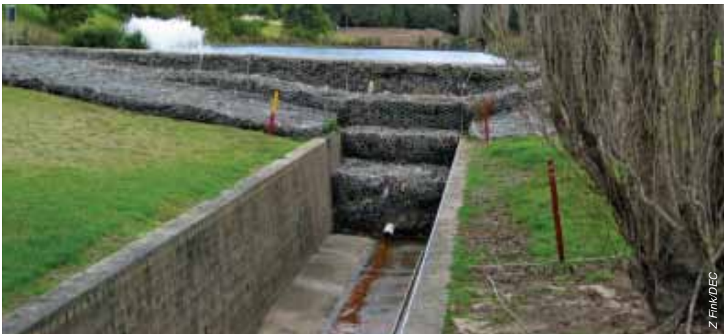
Weir at Bexley Golf Course (note spray from aerator)
