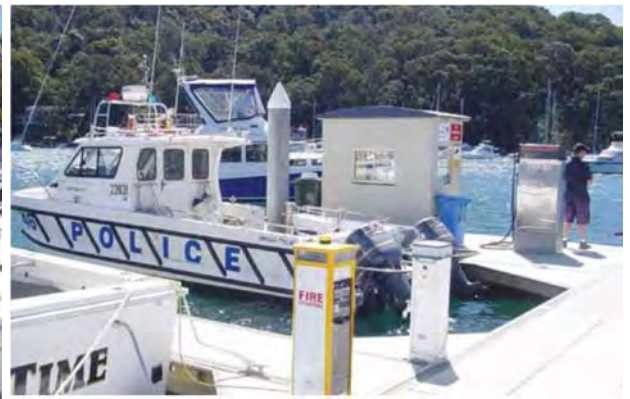
Photo G: View of a cabinet housing a fire extinguisher. A services pedestal is also visible behind the cabinet.
