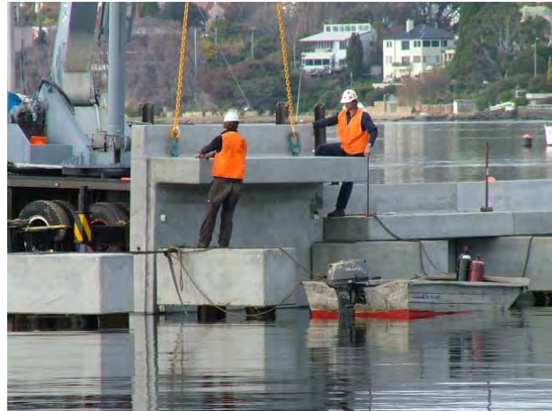
Photo B: Construction of fixed panel wave attenuator – showing fixed panel being positioned onto pile caps
