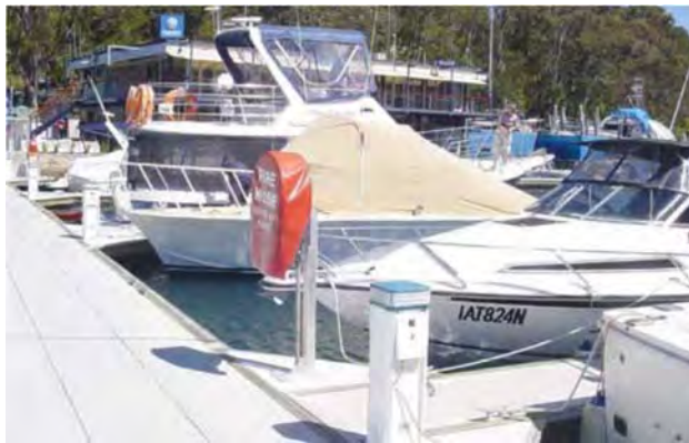
Photo E: View of a typical services pedestal within a floating marina. A fire hose reel is also visible behind the services pedestal, with a red cover.
