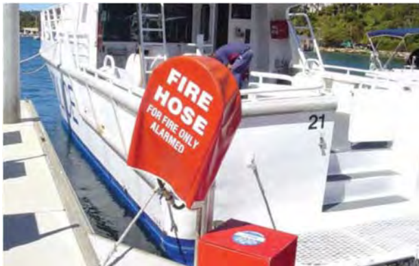
Photo F: Example of a fire hose reel within a floating marina
