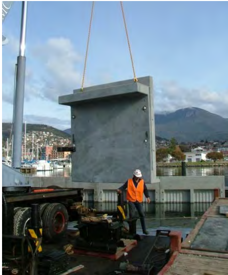
Photo A: Construction of fixed panel wave attenuator – showing fixed panel being lifted into place by floating crane.
