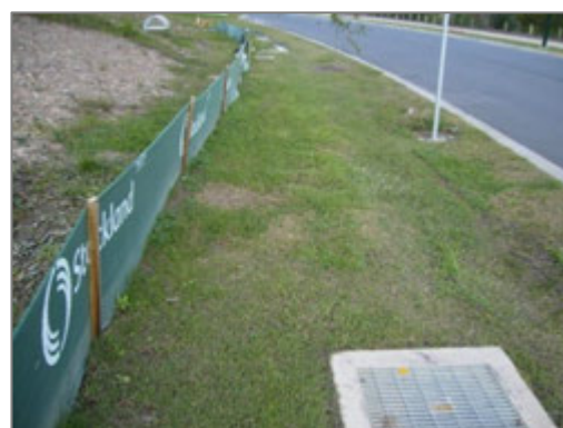
Example of Sediment Fence on a Construction Site
