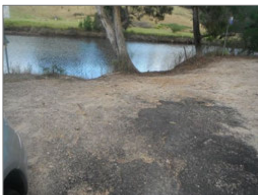
Foreshore Erosion on Yowaka River from shoreline fishing
