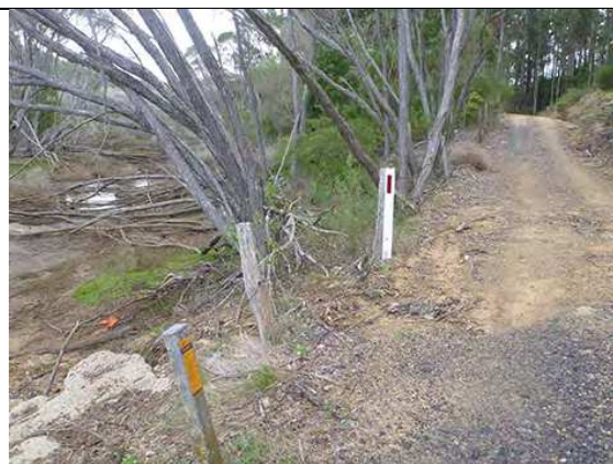
Figure B8 Inadequate road runoff controls has resulted in moderate erosion to Head of Cuttagee Road with some sediment depositing to estuary on western side ( left image ), and sediment also depositing to estuary on eastern side ( right image ).
