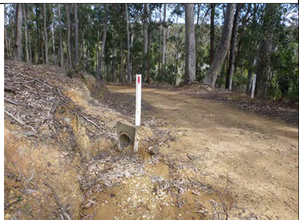
Figure B5 Erosion of roadside embankment on Head of Cuttagee Road adjacent to Lot 183
