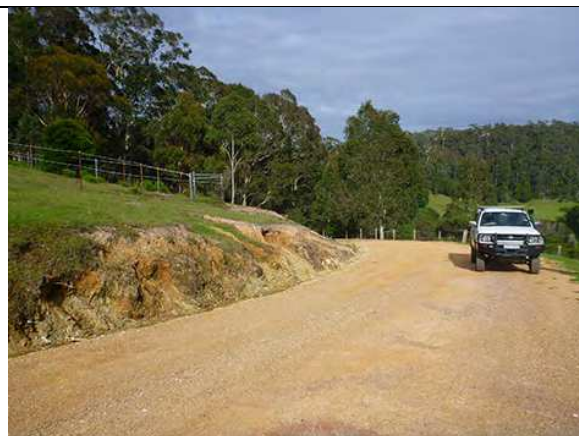
Figure B5 Erosion of roadside embankment on Head of Cuttagee Road adjacent to Lot 183
