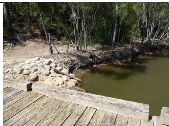
Figure B8 Inadequate road runoff controls has resulted in moderate erosion to Head of Cuttagee Road with some sediment depositing to estuary on western side ( left image ), and sediment also depositing to estuary on eastern side ( right image ).
