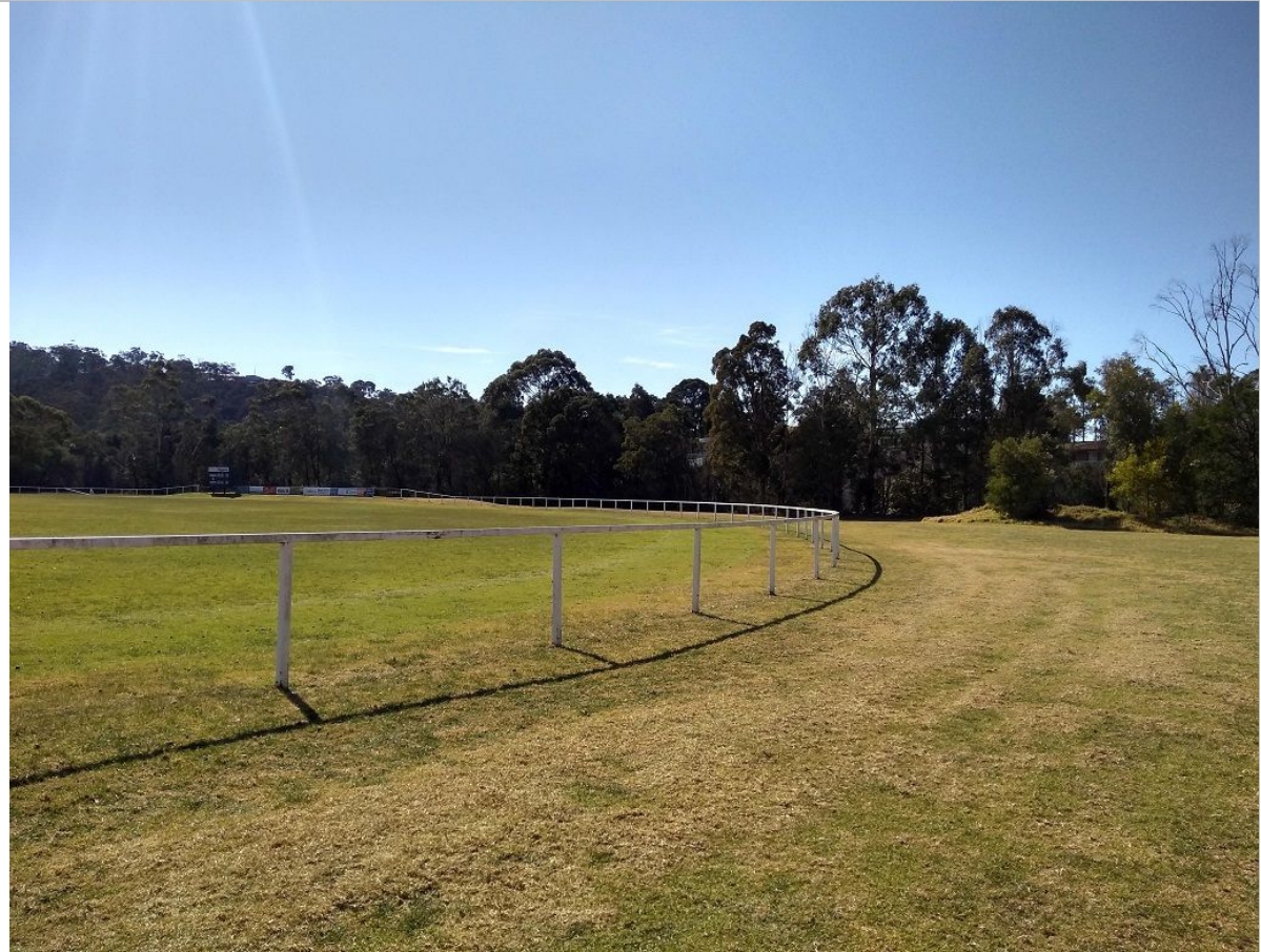
Steel rail fence along perimeter of playing field. Electrical conduit to be placed underground 4500mm from fenceline.
