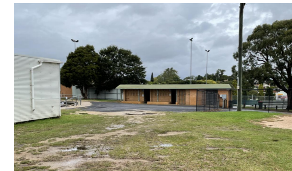
EXISTING TOILET BLOCK FROM CARP STREET
