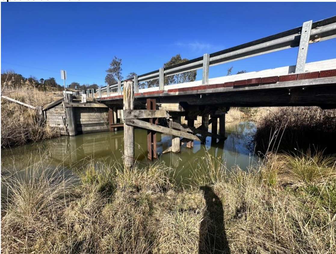
Photo 4, Underside of Katchencarry Creek Bridge, instream pier to be removed.
