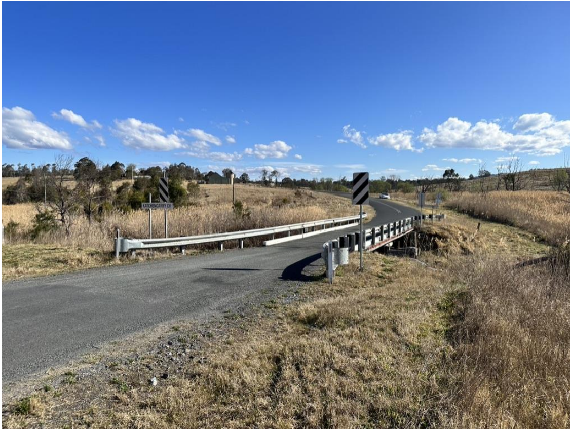
Photo 1, Katchencarry Creek Bridge from northeast side.
