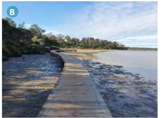
THE EXISTING BOARDWALK IS APPROXIMATELY 1.5M WIDE WHICH CREATES SOME CONFLICT WHEN PASSING WHEELCHAIRS, PRAMS, OR EVEN DOGS ON A LEAD. HOWEVER, THE NARROW WIDTH IS CHARMING, UNOBTRUSIVE, AND VISUALLY CONNECTS PEOPLE TO THEIR SURROUNDINGS. IT IS PROPOSED THAT THE BOARDWALK IS WIDENED FROM 1.5M TO 2.0M WITH KICK RAILS TO ALLOW EASIER PASSING BUT TO STILL RETAIN THE VISUAL CHARM AND CONNECTION TO THE LANDSCAPE.
