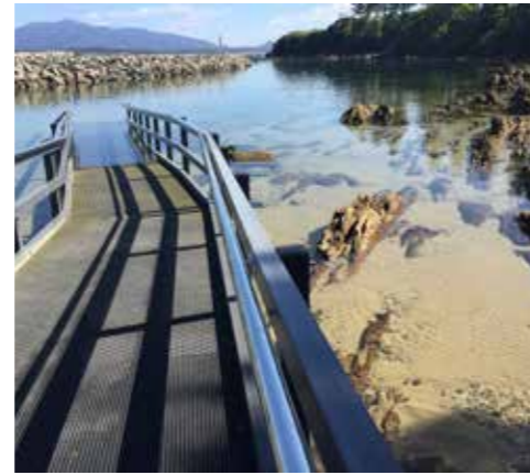
Accessible water ramp
