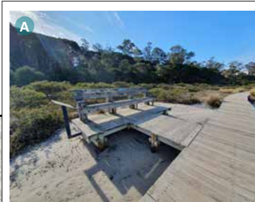
EXISTING BREAKOUT SEATING PROVIDES SPACE FOR VISITORS TO REST AND TAKE IN THE LAKE VIEWS AS WELL AS READ INTERPRETATIVE SIGNAGE. MORE SEATING SIMILAR TO THIS TO BE PROVIDED ALONG THE LENGTH OF THE BOARDWALK.
