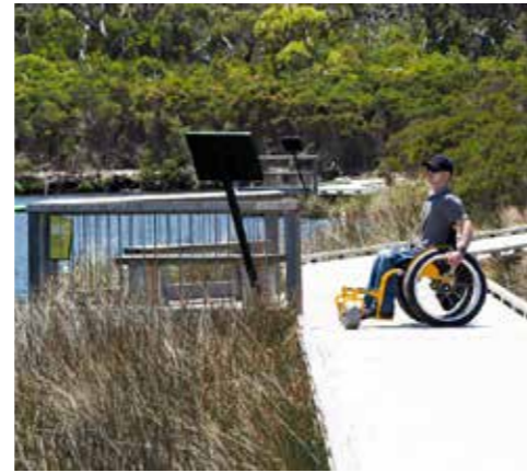
Boardwalk wider with kick rail and seating nodes off to the side
