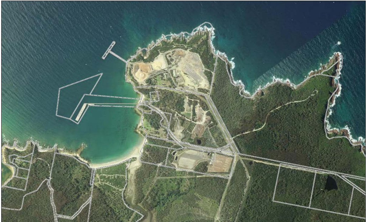
Figure 2: Aerial image of Edrom. Source: SIX Maps
