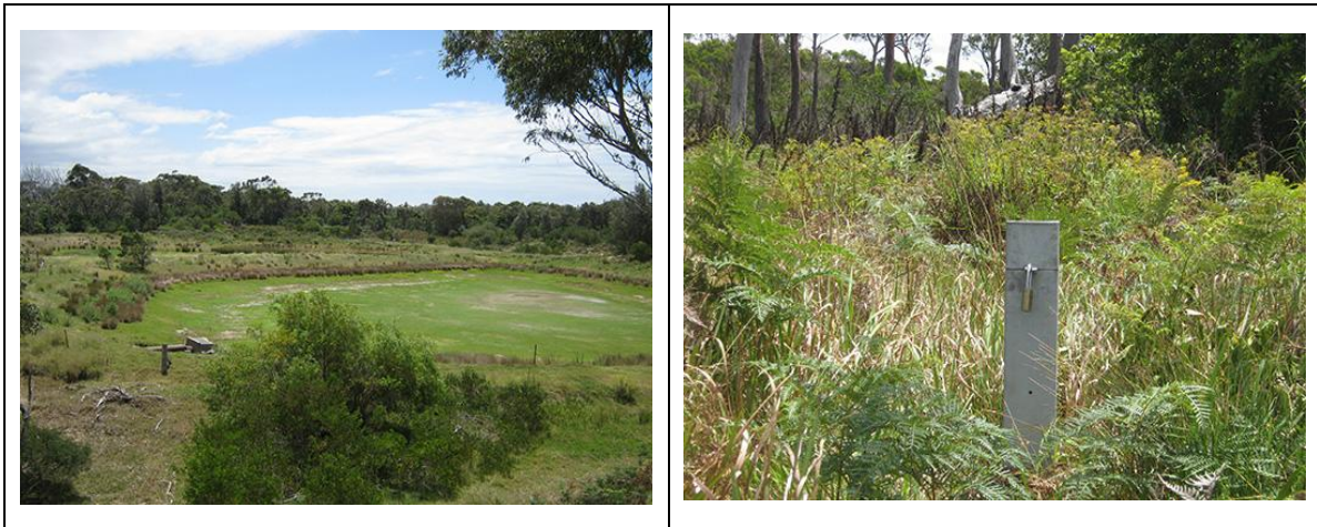
Figure 10. Merimbula STP dunal exfiltration ponds - empty ( left image ); monitoring bore BH10, adjacent to the ponds, used to measure groundwater levels for ponds usage ( right image ).
