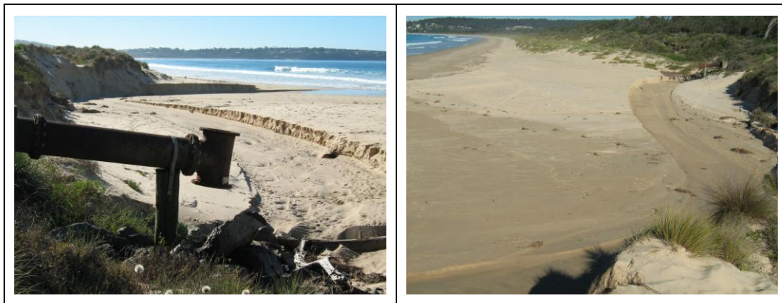
Figure 9. Merimbula STP ocean outfall pipe terminating in the foredunes ( left image ); discharged effluent flows across the beach to the ocean as evidenced by scouring of beach sands ( right image ).
