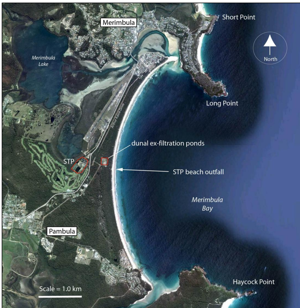
Figure 1. Location of the Merimbula STP and beach outfall.
