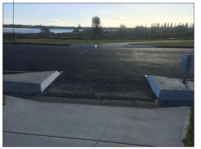
PEDESTRIAN CROSSING LAMONT STREET BERMAGUI CROSSING IN ACCORDANCE WITH RMS TECHNICAL DRAWING T000711 BLISTERS IN ACCORDANCE WITH RMS TECHNICAL DRAWING T000962
