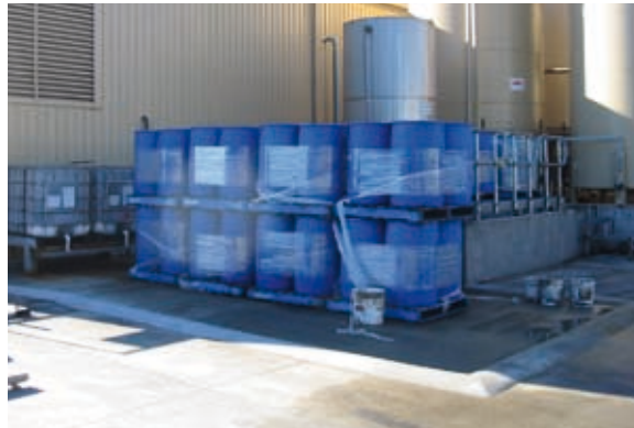
Above: Speed humps can be a useful form of secondary containment, especially over driveways.
