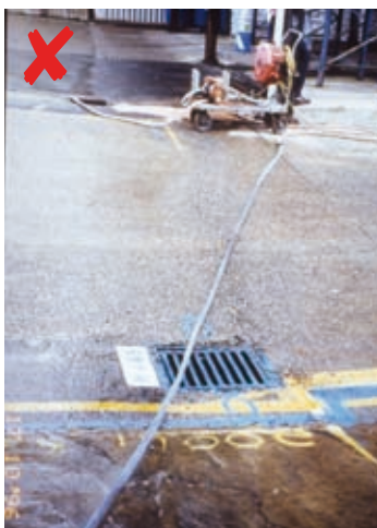
Above left: Hoses, pipes and taps can rupture or fail for a variety of reasons. This activity poses a high risk of water pollution because there is no method of secondary containment. Above right: Decanting smaller containers requires planning and management.
