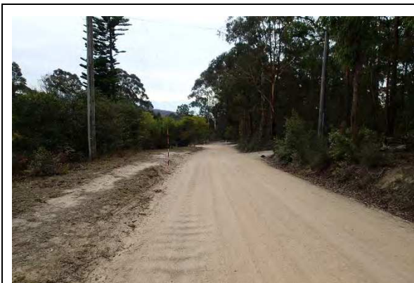
Plate 5. View north along road showing cutting and imported road base.
