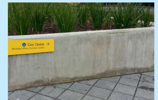
Concrete retaining wall
