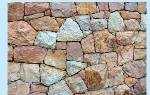
Stone retaining wall
