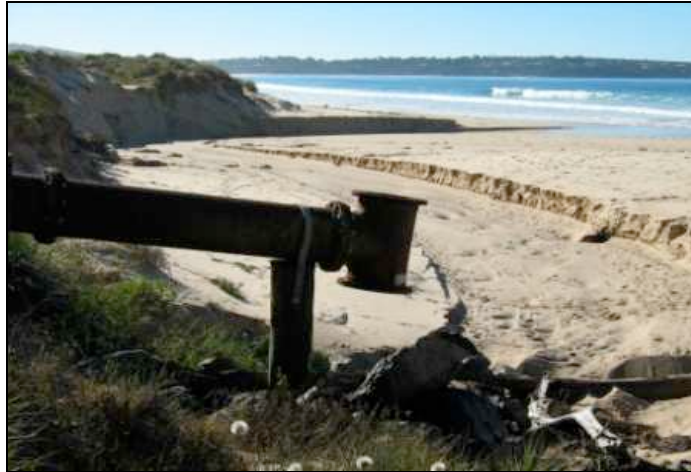
Figure 10: Existing shore based ocean outfall
