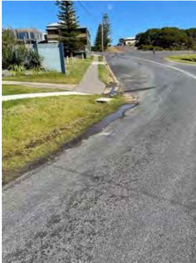
Figure 2.6 – Typical stormwater treatment within study area.
