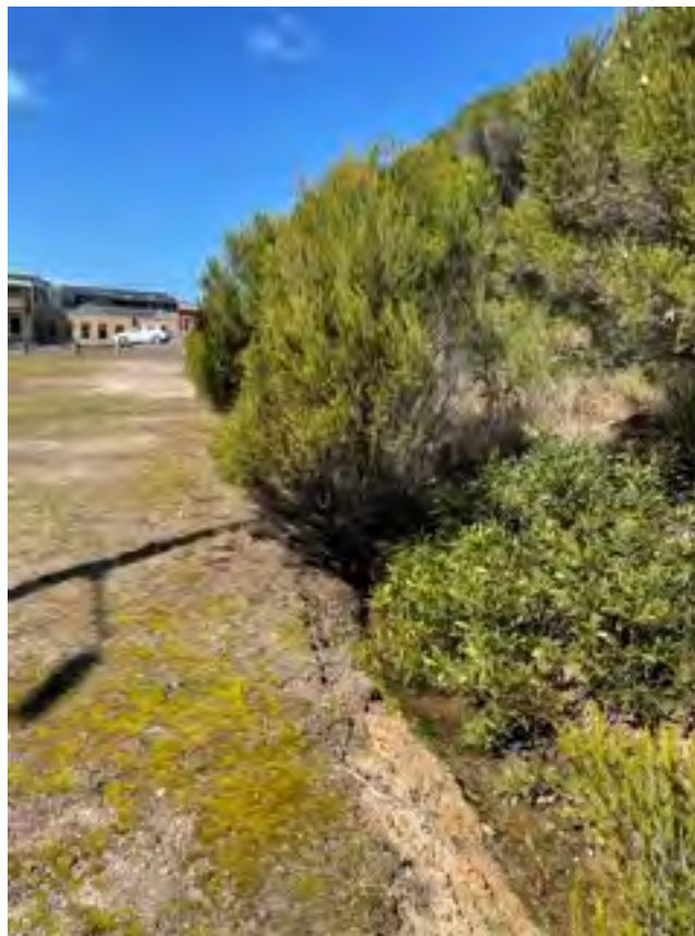
Figure 2.1 – Swale drain linking Service Road junction (hotel carpark) to Wharf Road.
