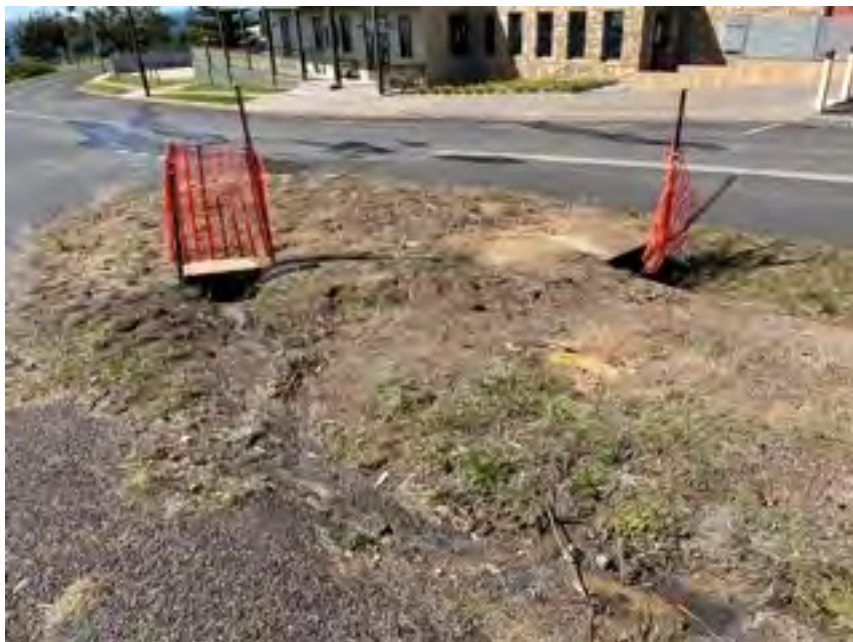
Figure 2.7 – Typical stormwater treatment within study area.
