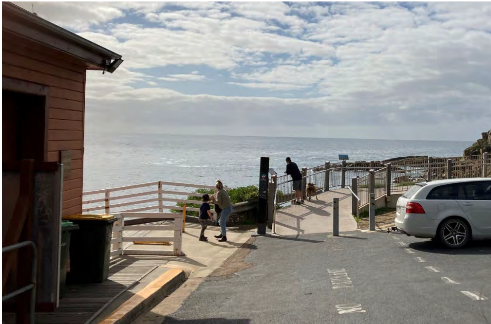
Figure 2.4 – Flush kerb at Wharf crossover directs stormwater down to retaining structure discharge as per Figure 2.3
