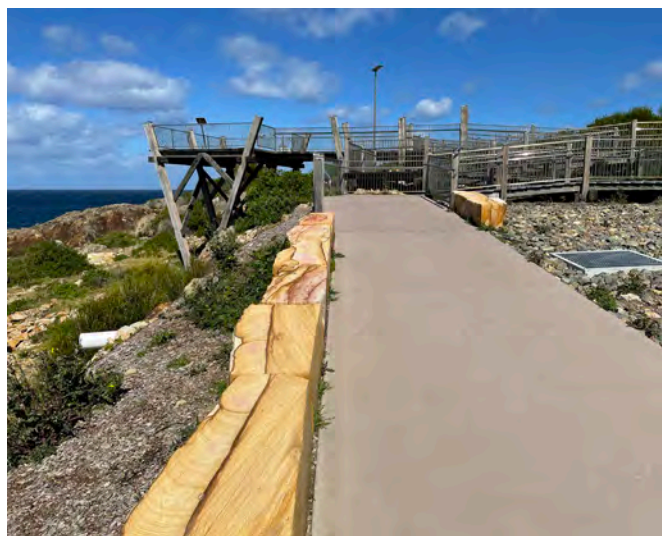
↑ Drainage pit and discharge to natural surface under path
