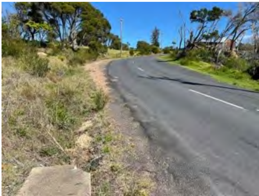
Figure 3.1 – Wharf Road (Looking South).
