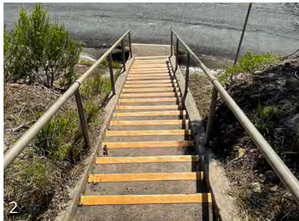
Stairs to the Wharf with appropriate safety elements while retaining landscape character
