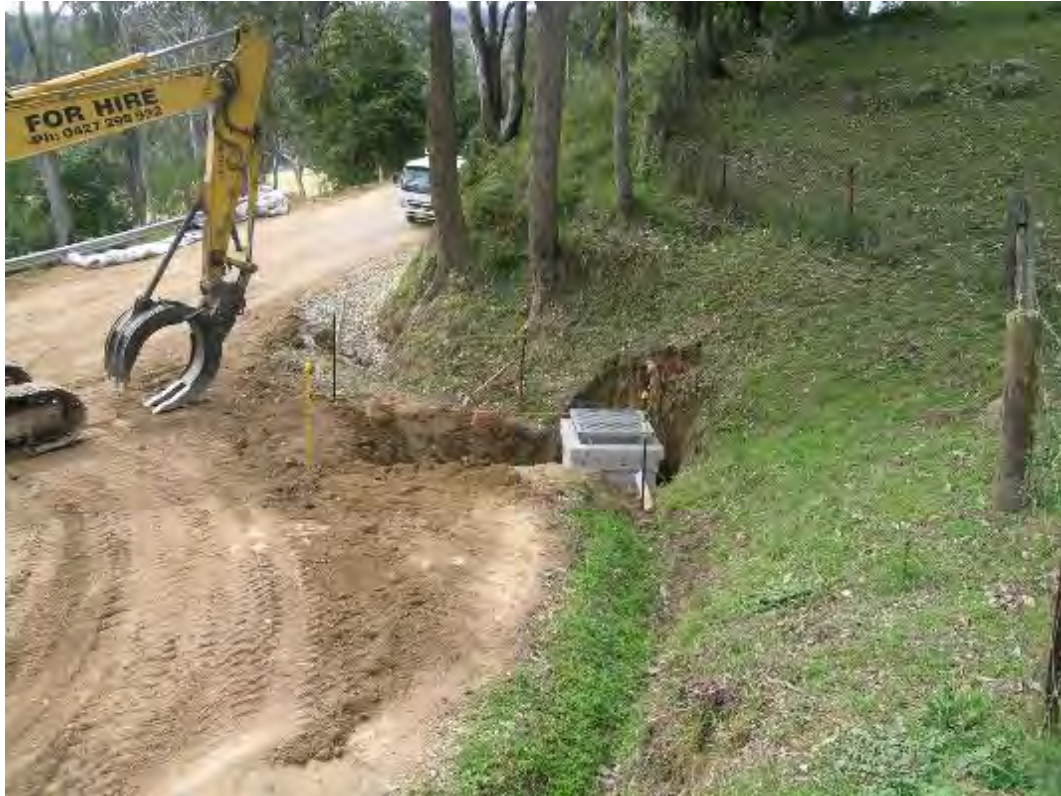
Photo 18: Installation of the second road drain (dated 22 August 2013).
