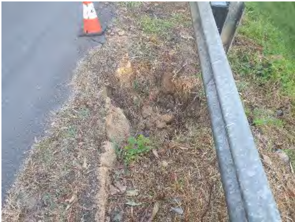
Photo 14: Close up photo of hole in the road shoulder between the road and steel guardrail (dated 10 August 2021).
