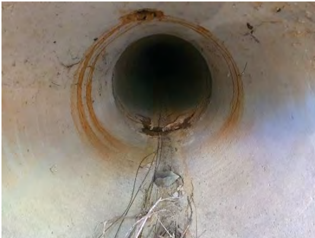
Photo 16: Close up shot of inside the northernmost culvert pipe, note slight damage in the pipe connection of the first pipe segment (dated 10 August 2021).
