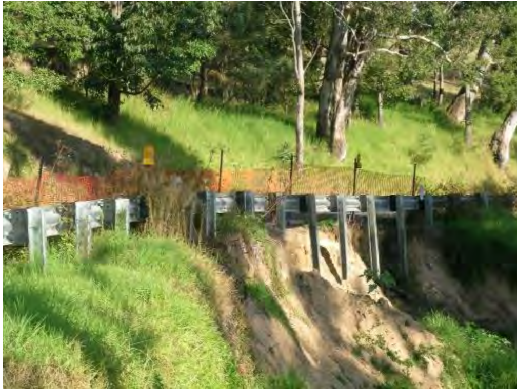
Photo 22: Road collapse behind and around the steel guard rail, noting the steep sloping embankment (undated).
