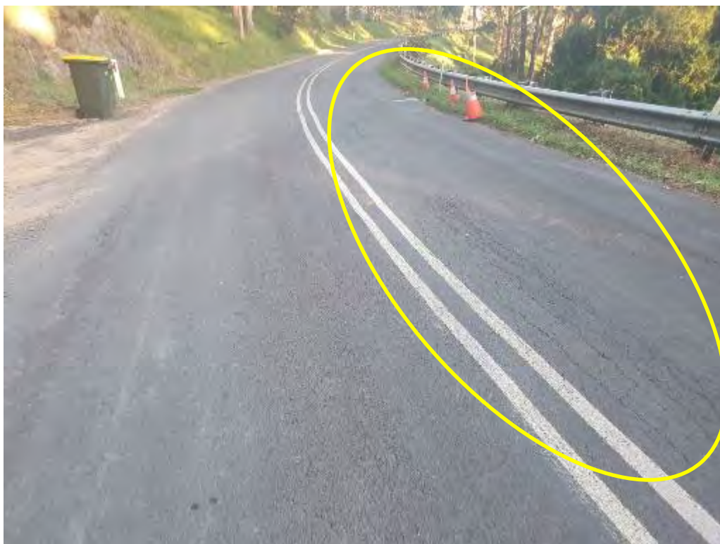
Photo 12: Approximate chainage CH770. Not tension cracks forming in the eastbound lane (downslope side). Areas of the eastbound lane are also slightly depressed (dated 10 August 2021).
