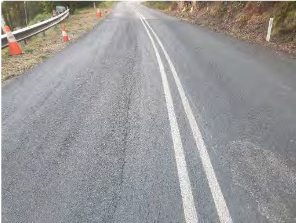
Photo 13: Looking east towards tension cracks in eastbound lane, nearby to the centreline (dated 10 August 2021).
