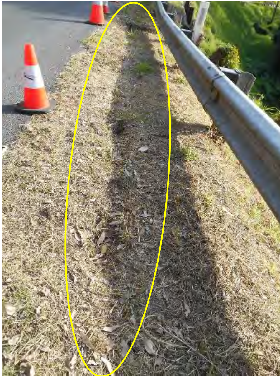
Photo 17: Close up photo of the tension crack in the road shoulder, several deep holes up to 100 mm deep are present and in some areas a step 50 mm in height has formed (dated 27 July 2021).
