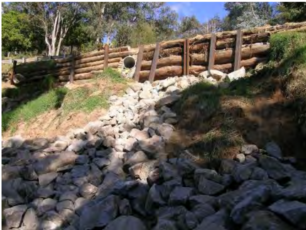
Photo 21: Looking up towards the restored roadside and two culvert pipes. Note erosion below the retaining way structure (dated 21 May 2010).
