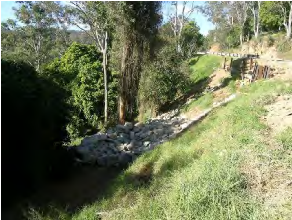
Photo 23: Rock filter dam at the base of the two culvert pipes (dated 21 May 2010).
