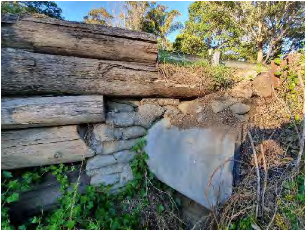
Photo 10: Close up shot of the area around culvert pipe outlet in the retaining wall (dated 10 August 2021).
