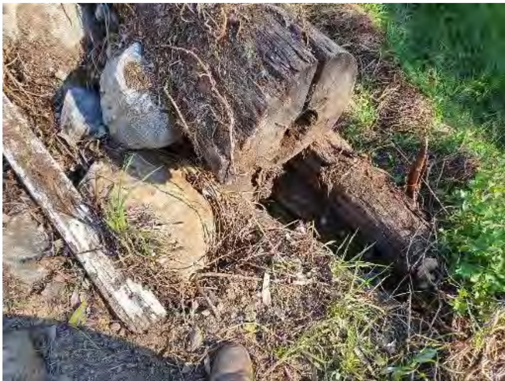
Photo 11: Close up shot of decomposing logs hollowing out from the centre. Note material washout behind the timber logs and backfill material consisting of large granodiorite boulders (dated 10 August 2021).
