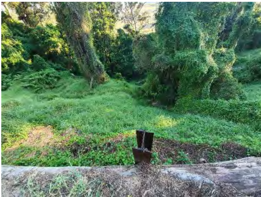
Photo 8: Standing on retaining wall looking down slope, note heavily vegetated fill batter (dated 10 August 2021).
