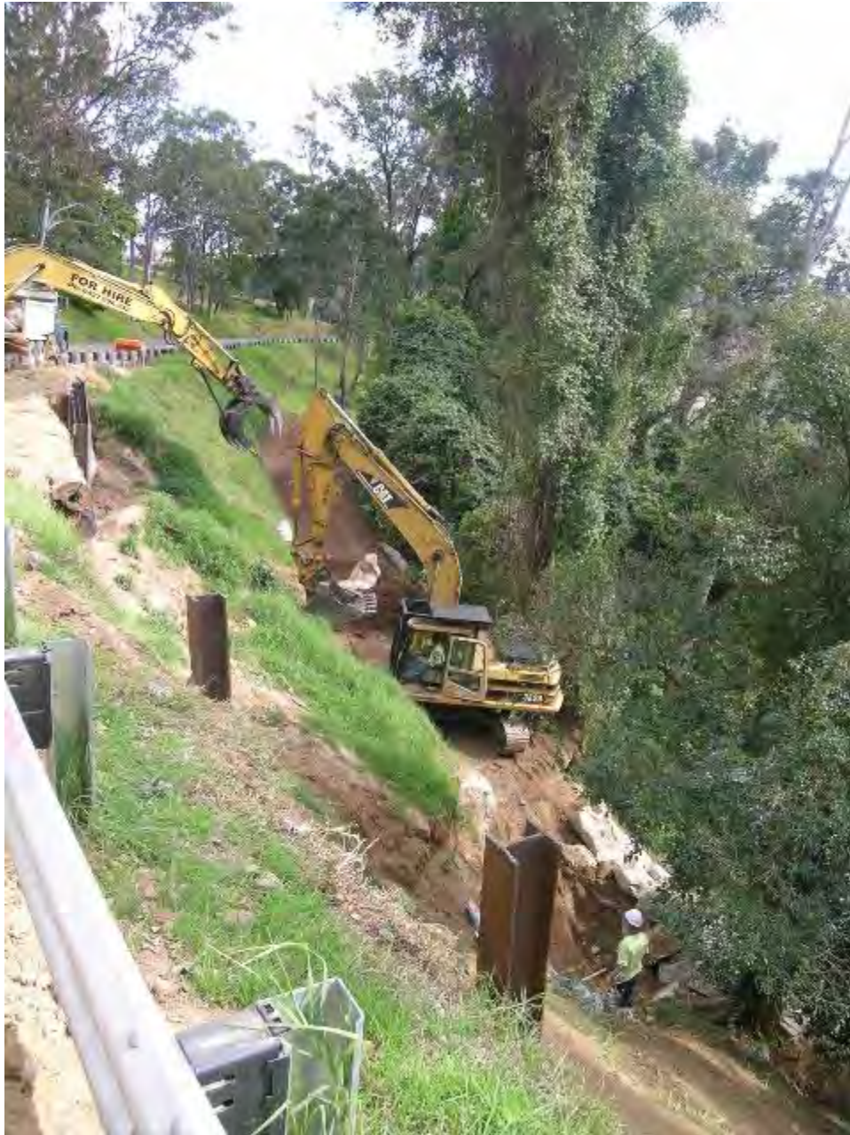
Photo 19: Looking down towards the construction of the filter dam adjacent to the road shoulder. Note the sloping embankment and erosion features below the steel guard rails (dated 19 August 2010).
