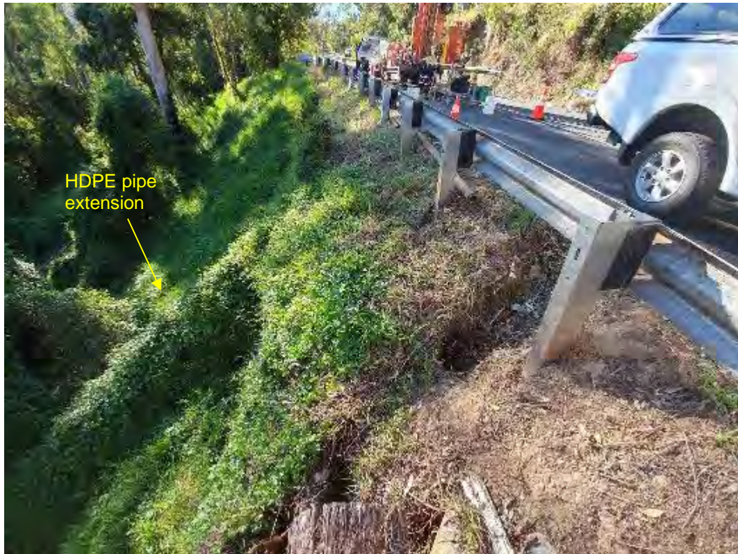
Photo 15: Looking east from the retaining wall, note holes and erosion in shoulder extending down behind the retaining structures (dated 10 August 2021).
